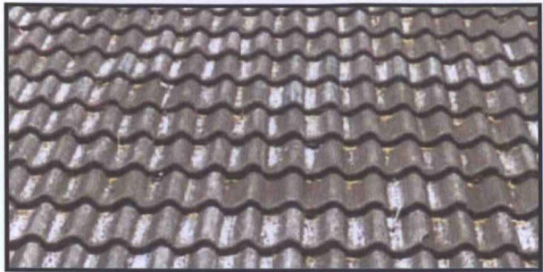
ROOF TILES: RETAIN EXISTING
