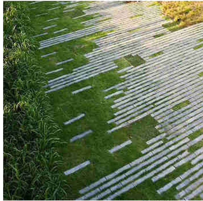
DRIVEWAY DETAIL - PERMEABLE
