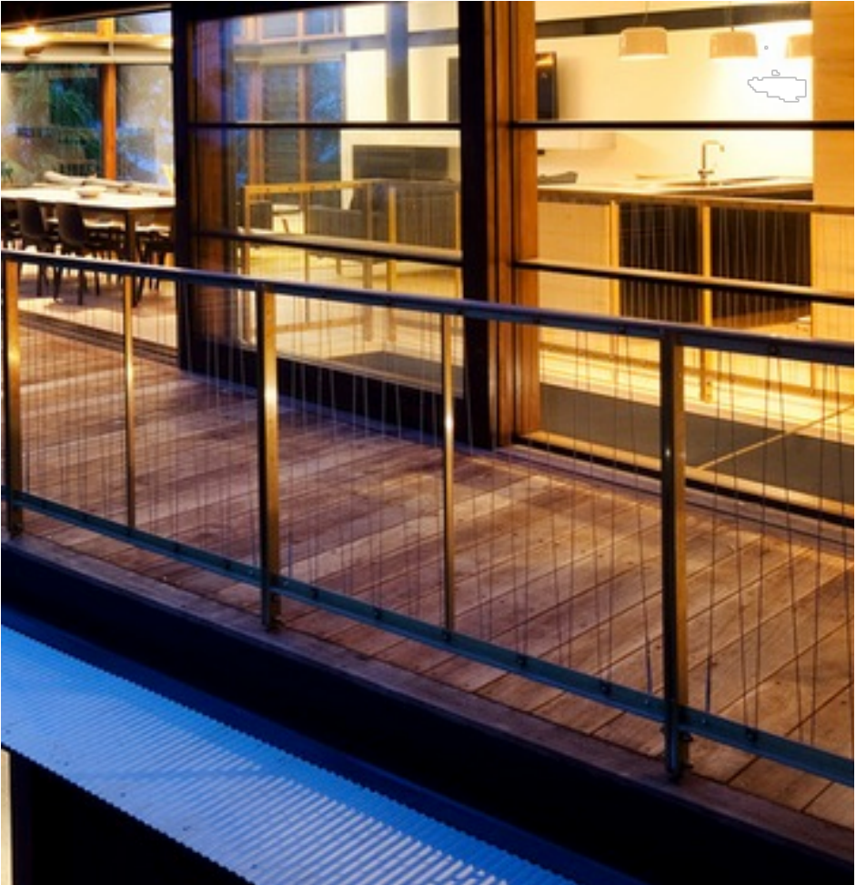
BALUSTRADE - STEEL WITH TIMBER RAIL
