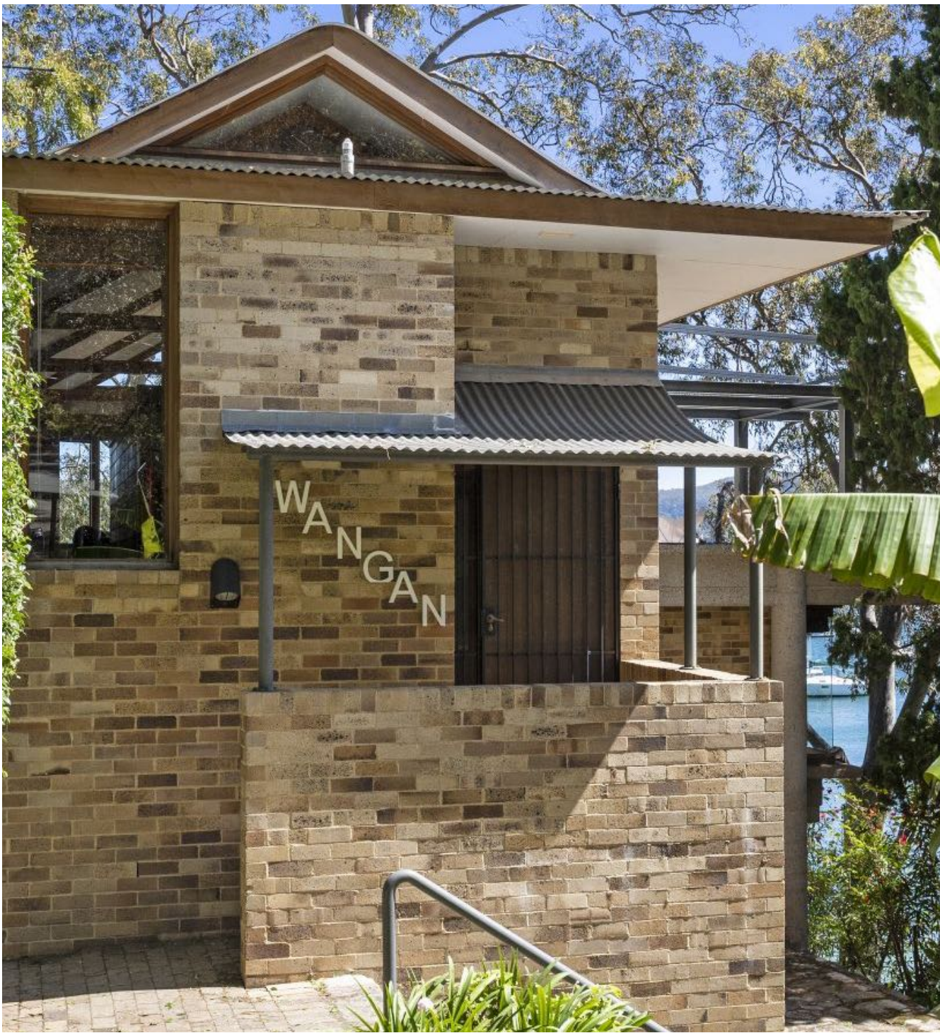
BRK1_ EXISTING BRICKWORK
