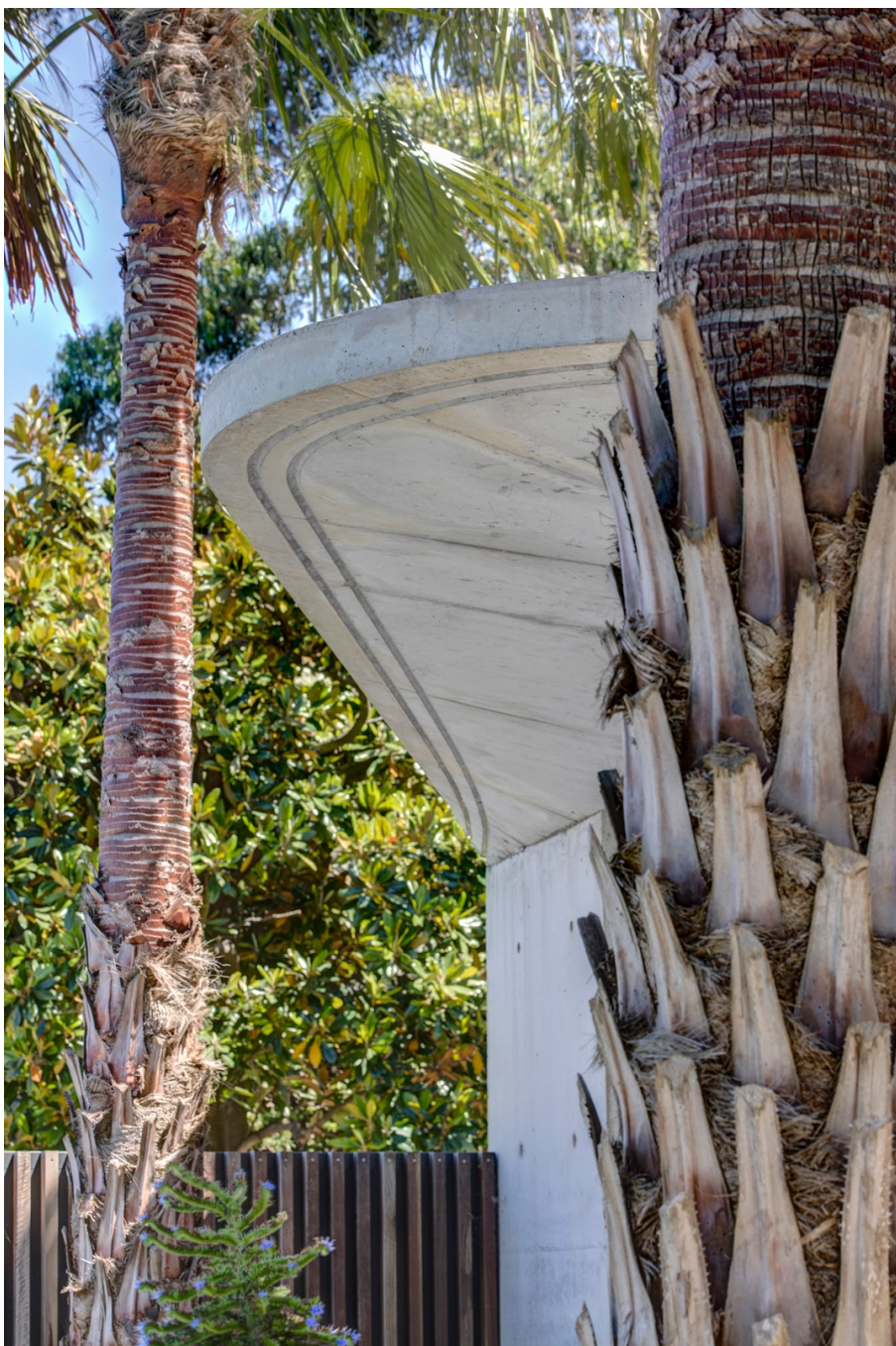
CONC2 _ NEW OFF-FORM CONCRETE
