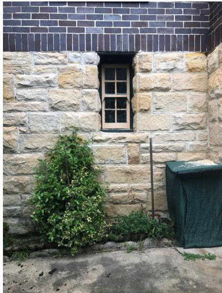
6 | Remediate and repair standstone and brick work was that remain
