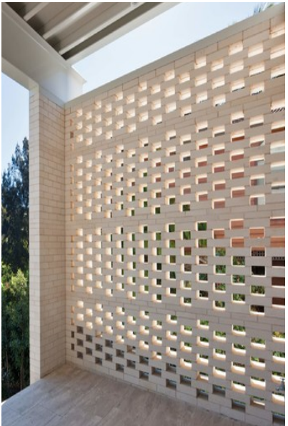
10 | Hit and miss brick screen Pattern to future detail.
