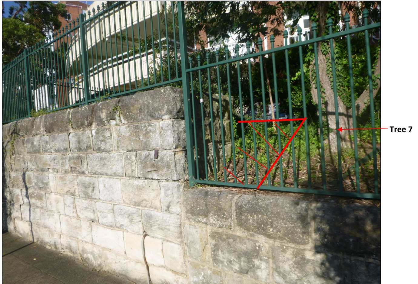
Photo A: Area where excavation may be required in the proximity of Tree 7.
