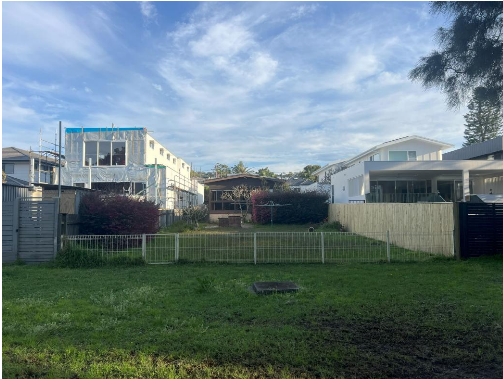
Photograph of the subject site from the rear pathway/reserve – 14 Stewart Avenue, Curl Curl
