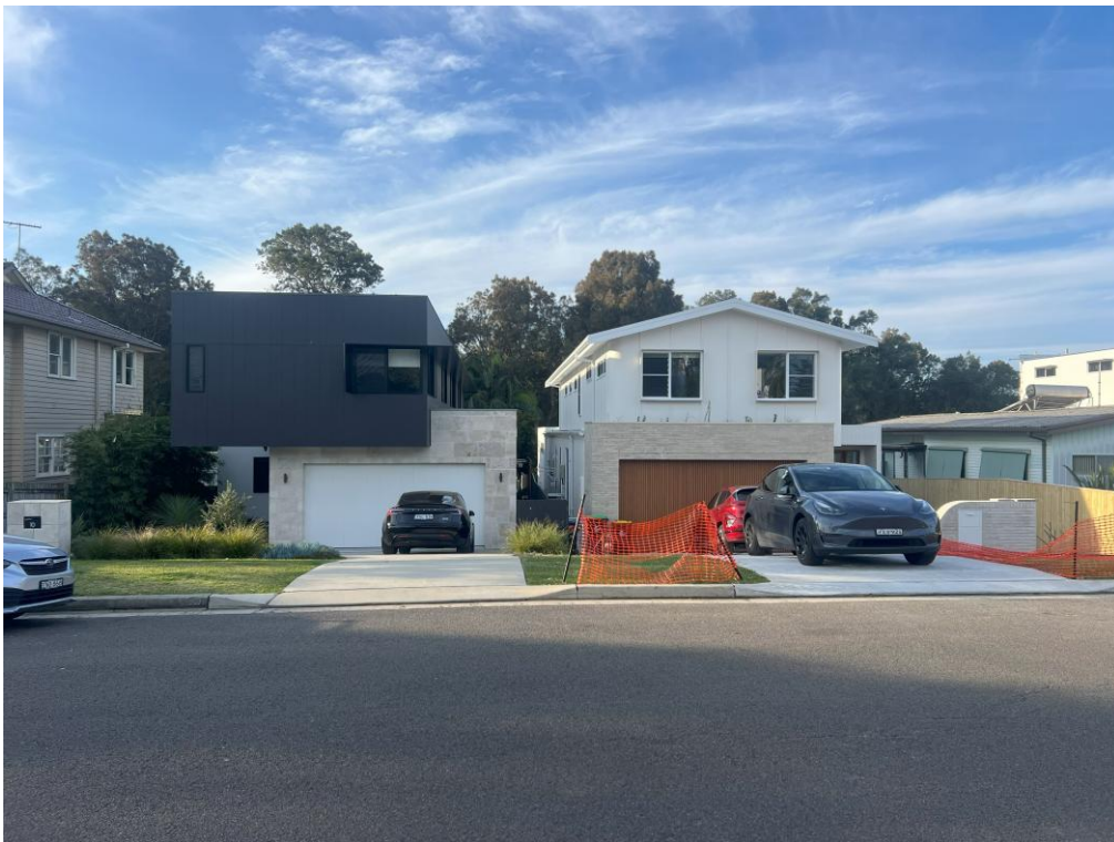
Photograph of 10 and 12 Stewart Avenue, Curl Curl – recently built modern dwellings
