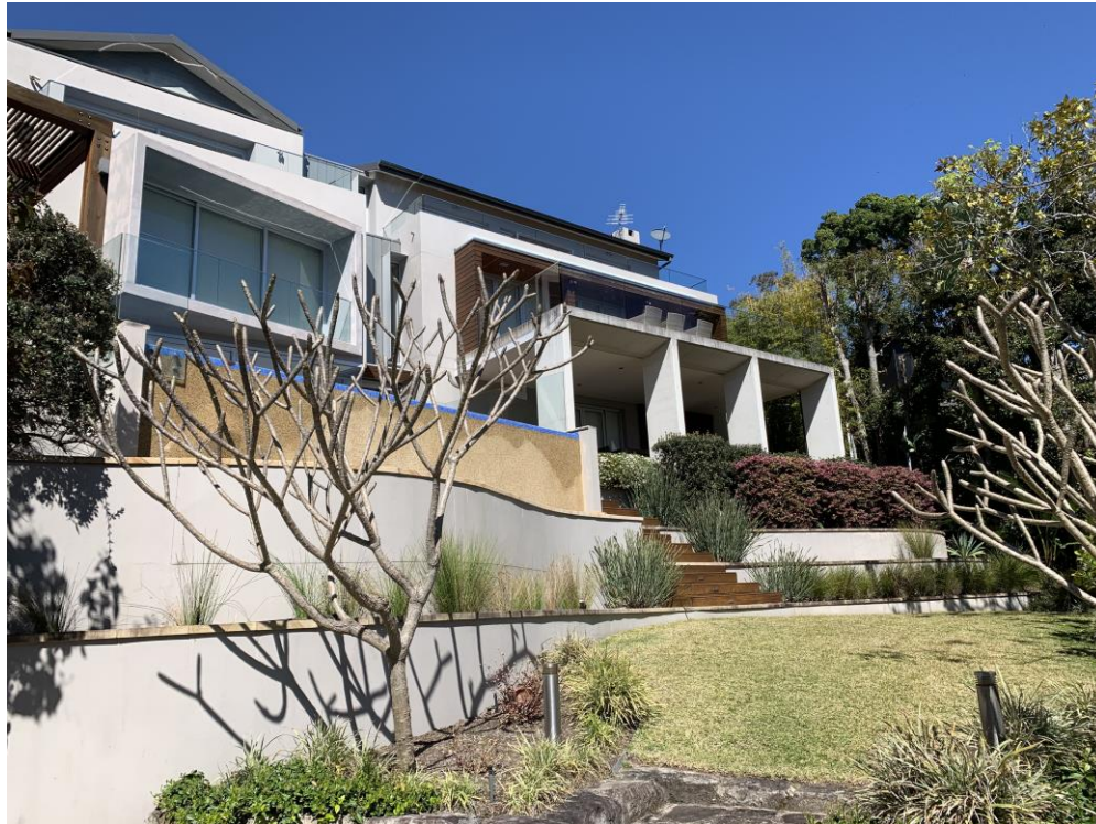
Fig 6: View of the northern elevation of the existing dwelling, looking south-east from the entry driveway from Mitchell Road
