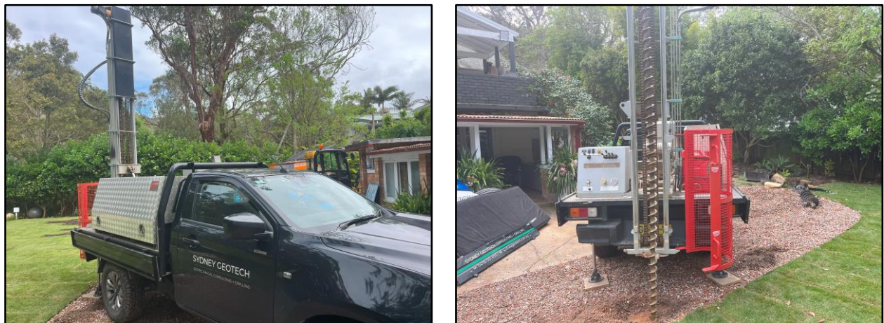
Figure 2 Ute Mounted Drill Rig
