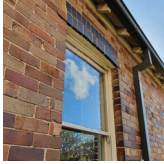
WINDOWS painted timber existing retained
