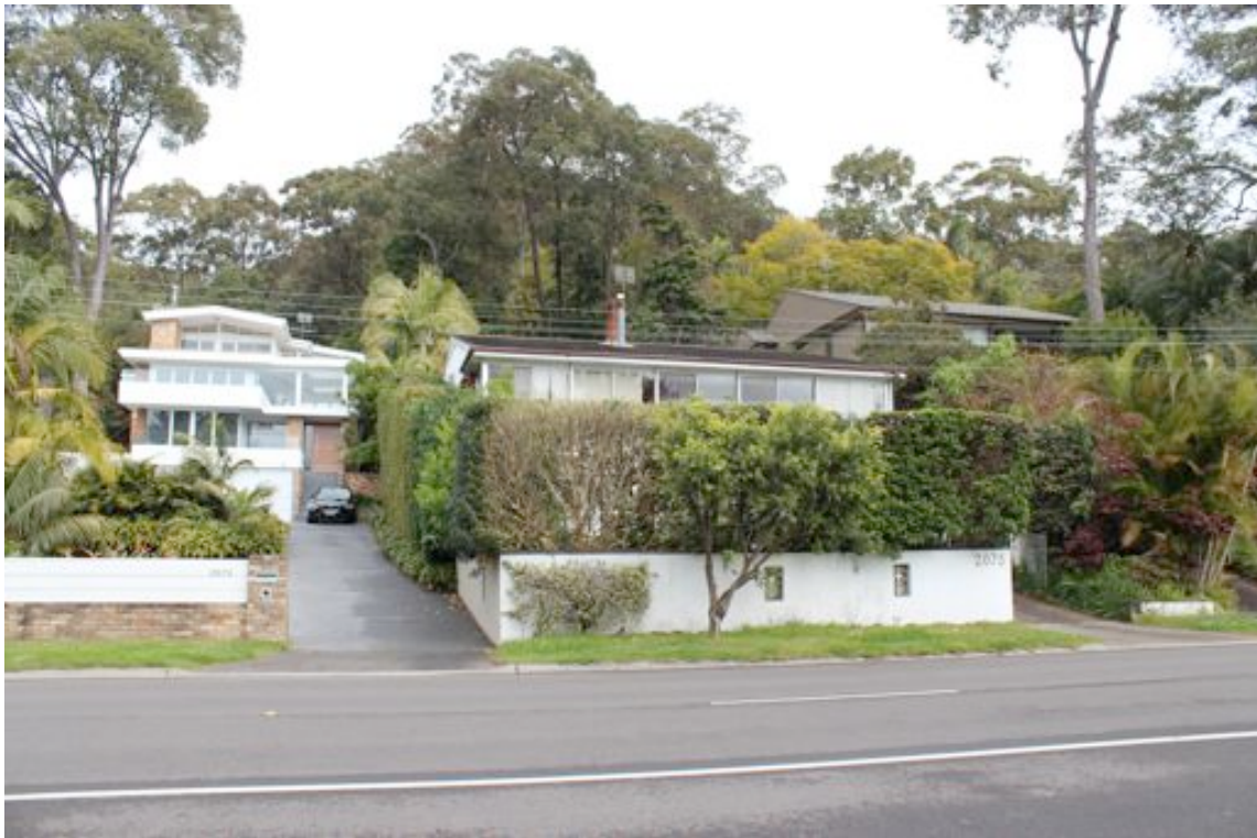
Subject site: No. 2075 Pittwater Rd showing existing dwelling
