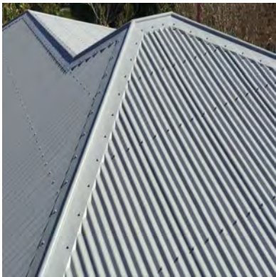
COLOURBOND METAL ROOF SHEETING. 'WINDSPRAY' OR SIMILAR
