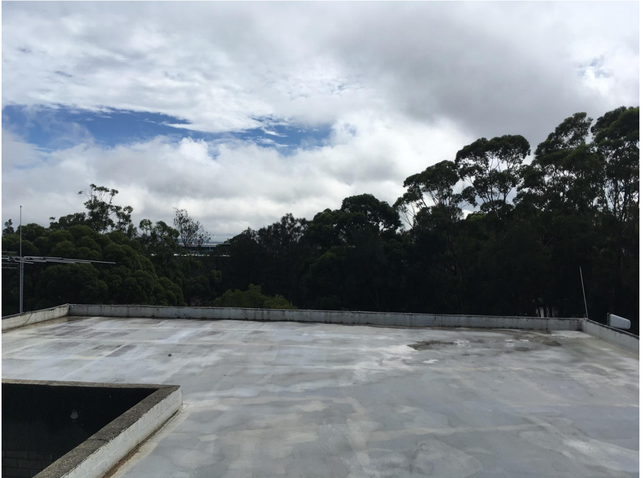
Photo 1. – Rooftop Site for Accommodating the Proposed Antennas
