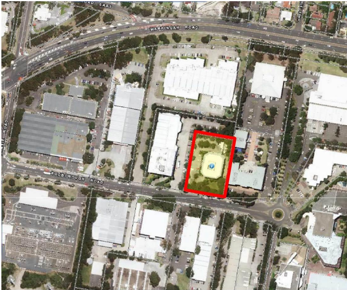
Figure 1. – National Playout Centre Building, Aerial View
