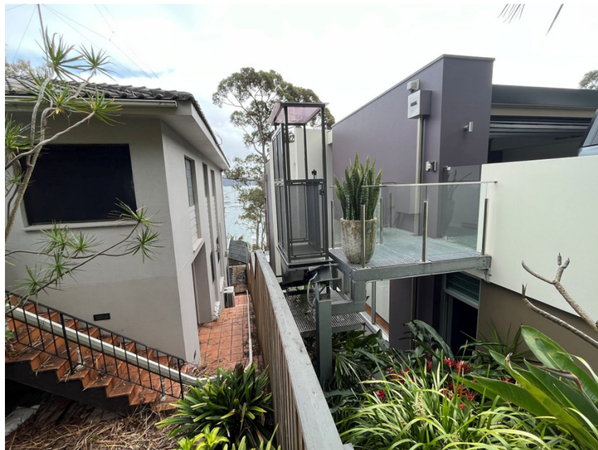
Photo 2: Elevated adjoining carriage and landing station & intended path of proposed Inclinor.
