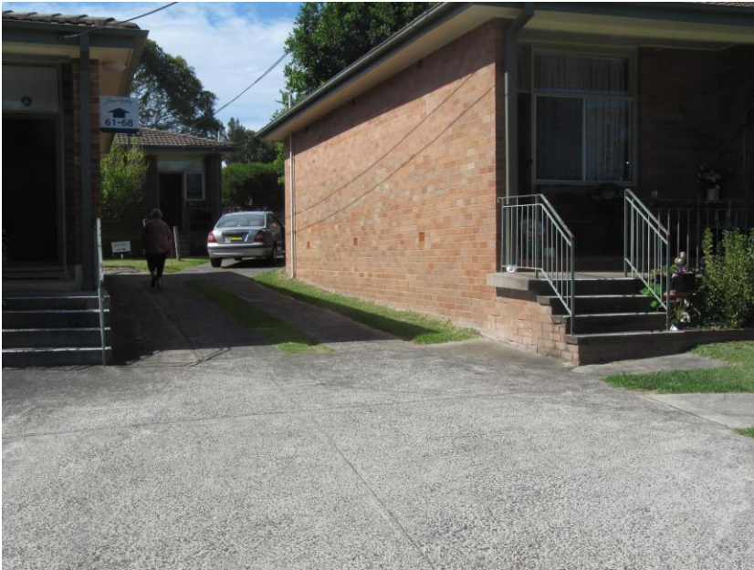
View 4 Driveway between Blocks 10 and 12 with Block 11 beyond
