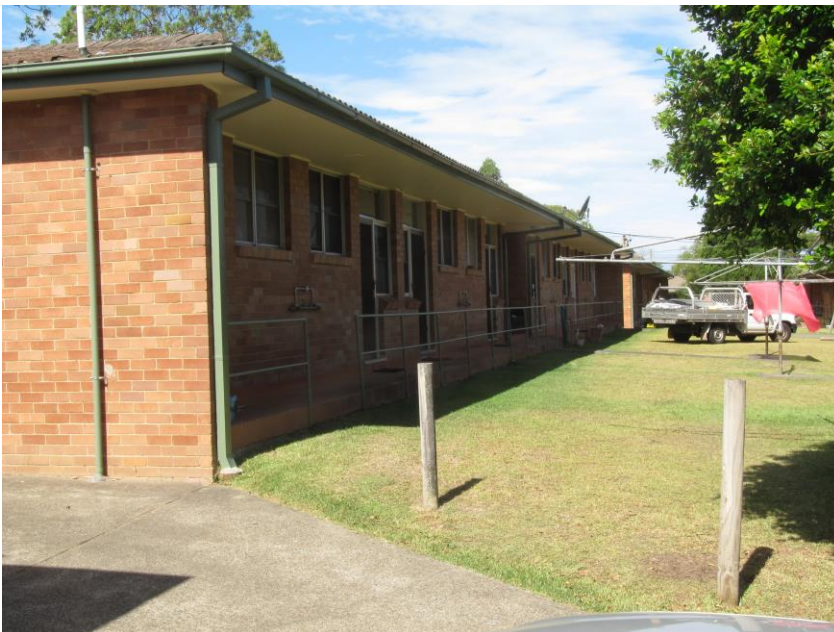
View 6 Looking eastward at the south-west corner of Block 9 which faces the internal courtyard (Block 7 and 11 similar)
