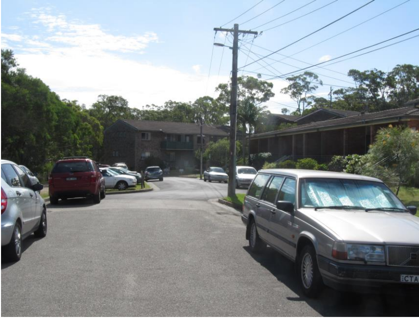
View 5 Looking westward along the internal road where Blocks 13 to 16 can be seen beyond
