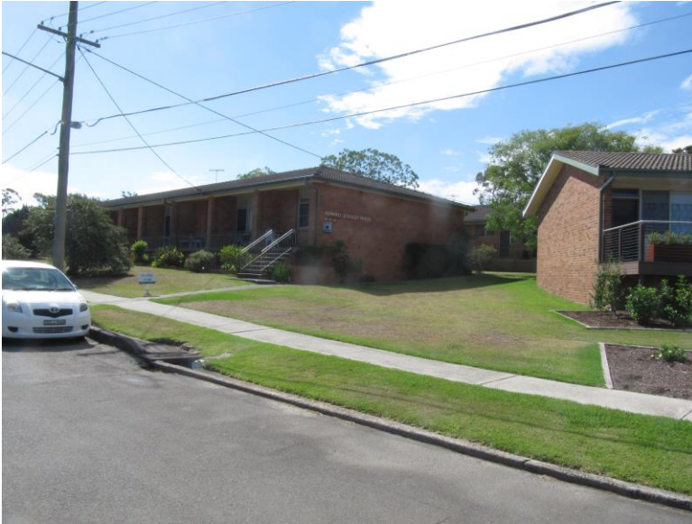
View 1 Eastern wall of Block 8 with Block 7 behind (southern end of Block 2 is seen on the right but is not part of this submission)
