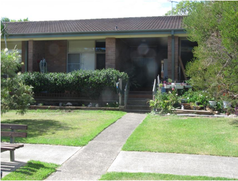
View 3 South wall of Block 10 facing internal roadway
