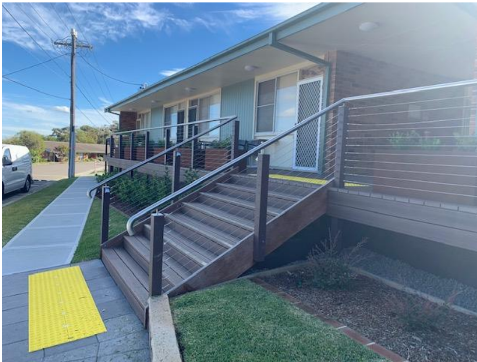
View 7 existing balustrade to Block 1
