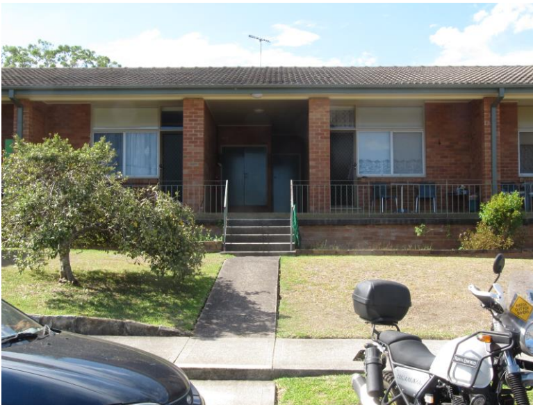
View 2 South wall of Block 8 facing internal road
