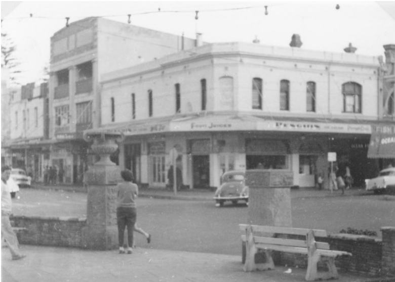
Figure 2.3 The former Ocean Beach Tea Rooms, c.1960, showing the early twentieth century extension on the east elevation and the broader visual impact of the replacement cantilevered awning upon the streetscape. Note the parapet has been removed, the exterior stripped of decorative details and the entire facade painted in white
