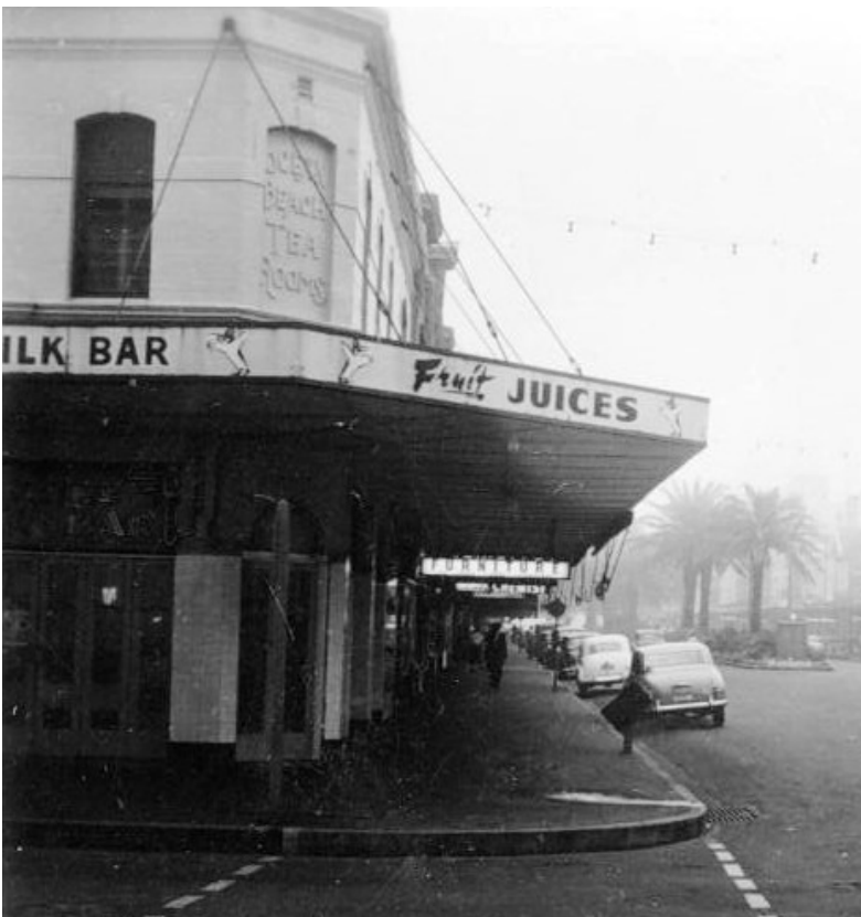
Figure 2.4 Detail of the exterior of the building. c1957, showing the tiled facade at ground floor level, the then-recent relocated entry and the altered window openings with unsympathetic aluminium folding doors.
