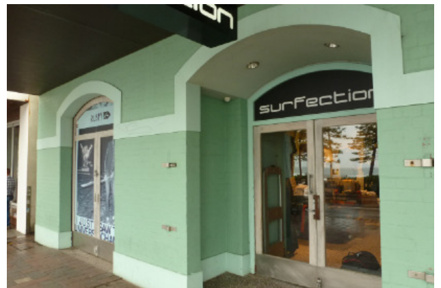
Figure 3.13 Detail of the reconstructed ground floor facade of The Corso elevation, showing new door and window openings and the insertion of contemporary materials as part of a retail fitout
