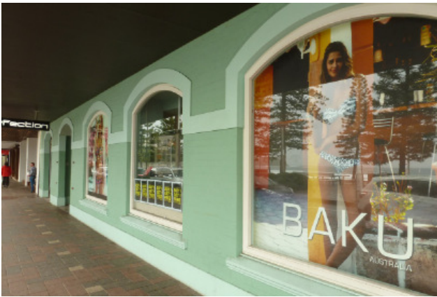
Figure 3.14 Reconstructed ground floor facade on The Steyne elevation
