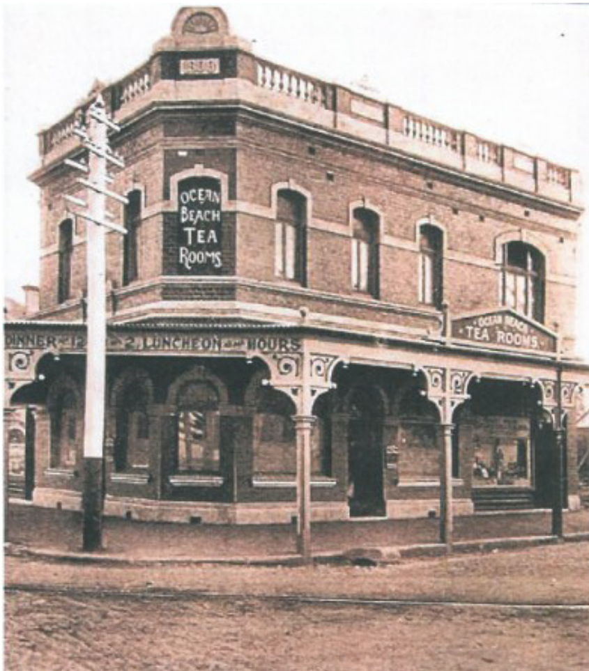
Figure 2.1 The Ocean Beach Tea Rooms as built in 1898, with its elaborate stop-chamfered timber posted verandah and decorative parapet
