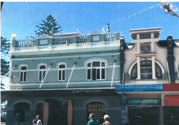
Figure 3.15 Detail of the reconstructed facade showing the interpretive parapet, mid-twentieth century replacement awning and roof top additions which are slightly visible above the parapet.
