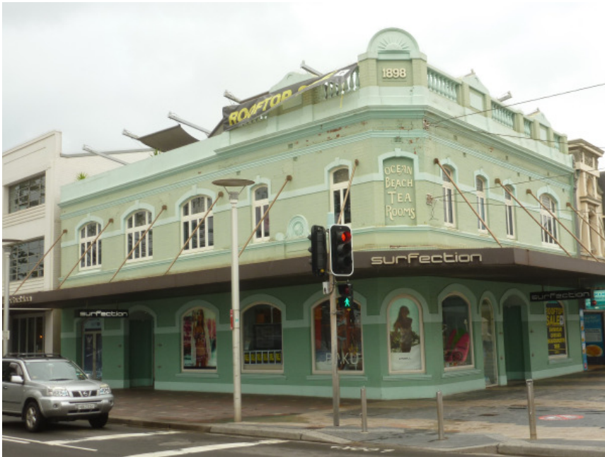
Figure 2.6 The Ocean Beach Tea Rooms current presentation, showing the extensive interpretive reconstruction works to the building's facade. Note the altered fabric to the window and door openings, and the mid-20C corner entrance has been relocated back to the original entry on The Corso. A more modest parapet was constructed to interpret the original, with the overall scale of works seeking to alleviate the heavily degraded fabric and improve the presentation of the building.
