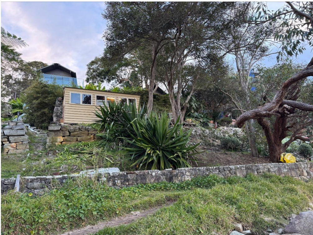
Photograph of the existing boatshed and retaining wall from lower level of site
