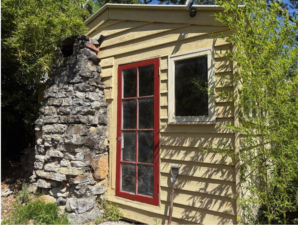
Photograph of the existing boatshed from the east with chimney to be retained
