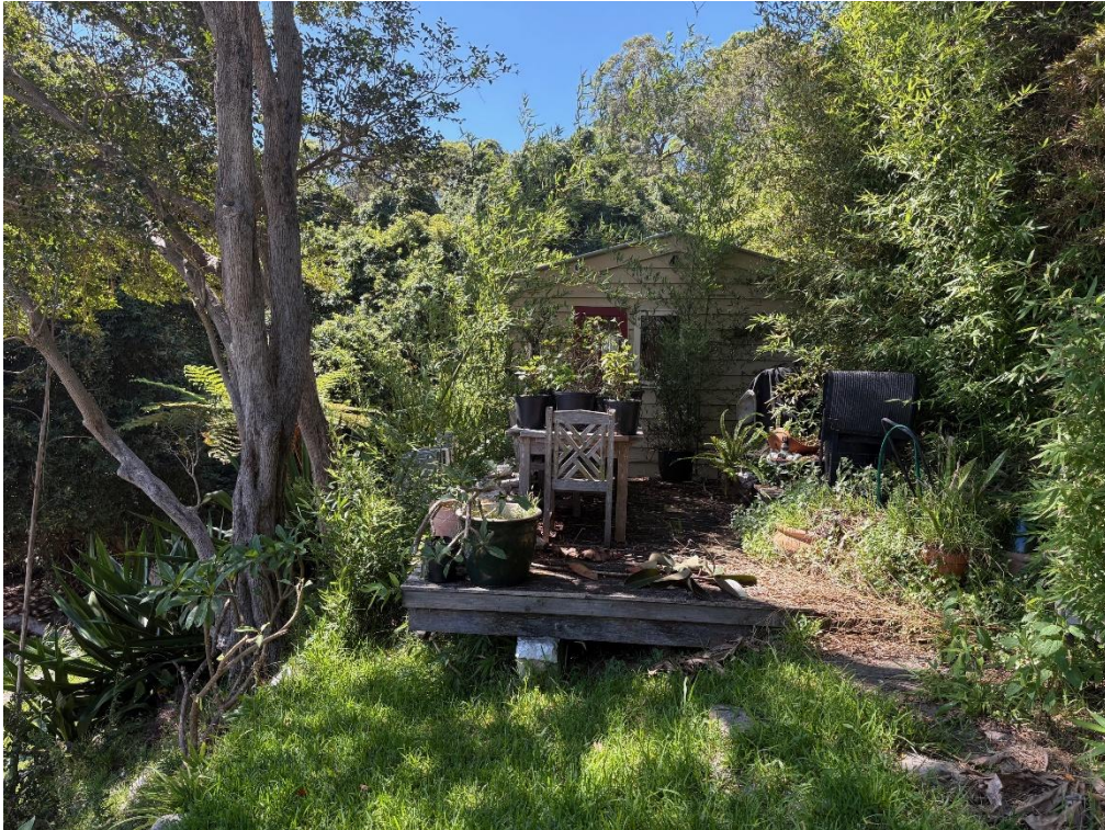
Photograph of the existing boatshed and decking
