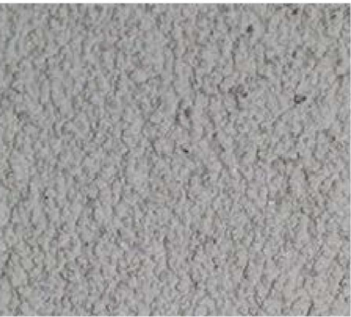
EXTERNAL RENDERED FOAM CLADDING - COLOUR TO MATCH EXISTING
