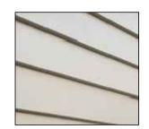
External cladding to match existing in profile Use "James Hardie - Axon" cladding as an alternative if original cladding cannot be matched.
