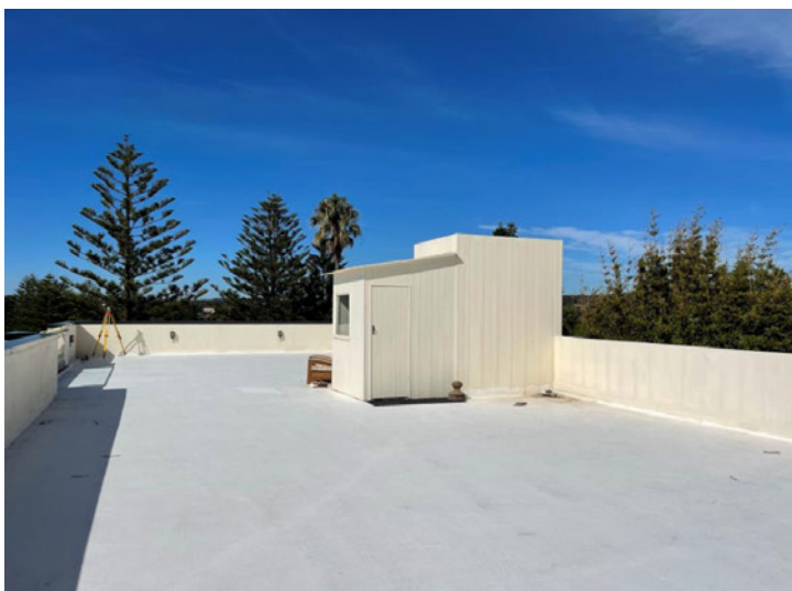
Current lift shaft and external shelter
