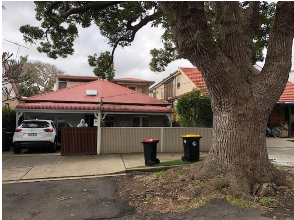
Figure 4. The existing semi-detached dwelling, looking north from Pacific Parade
