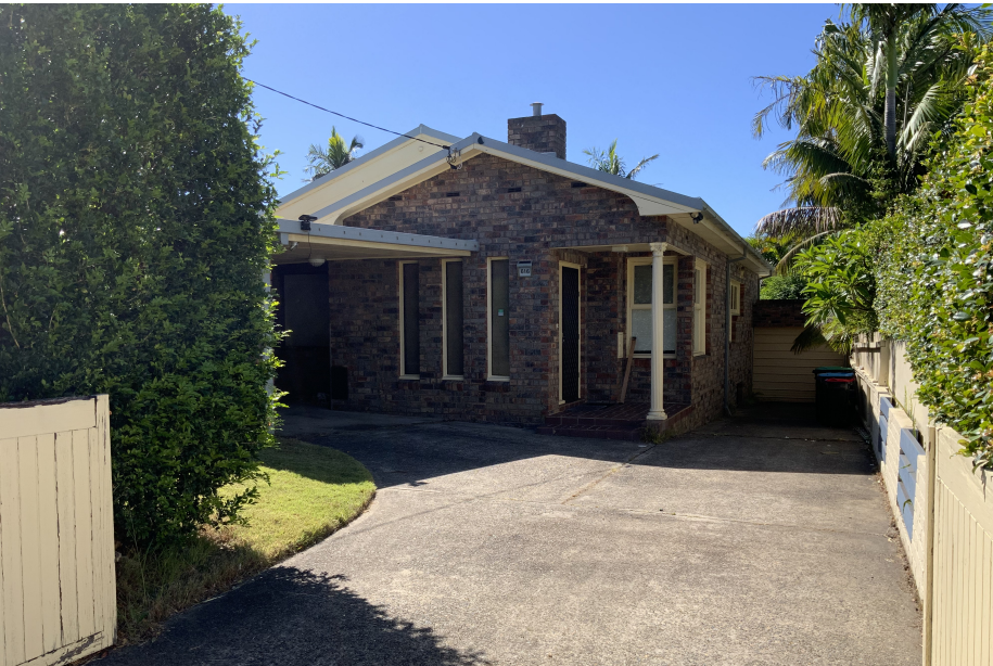
PHOTO OF NEIGHBOUR #616 SHOWING A CARPORT IN FRONT OF THE BUILDING LINE
