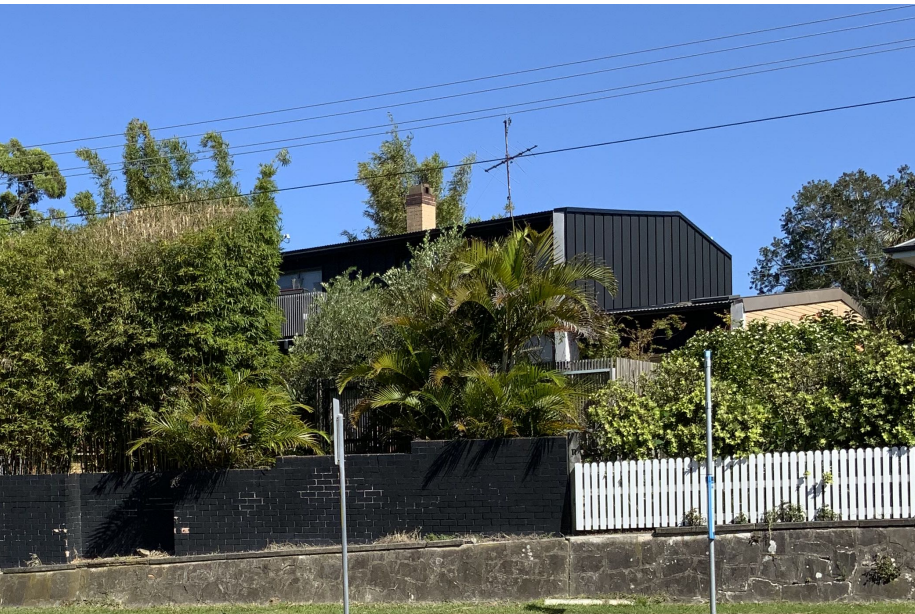
PHOTO SHOWING NEIGHBOUR #749 ACROSS THE ROAD FROM THE DEVELOPEMET SITE
