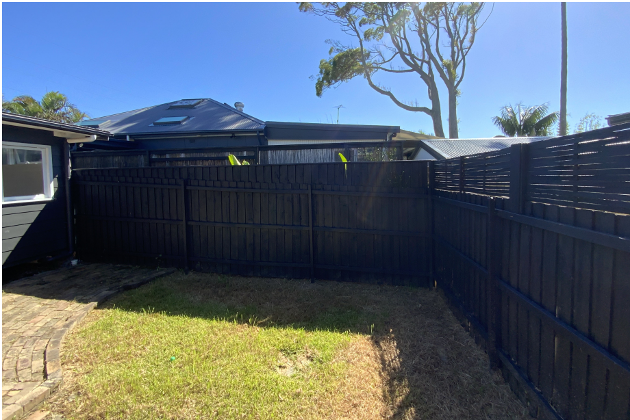
PHOTO OF EXISTING BACKYARD AND NEIGHBOUR #620 BEHIND
