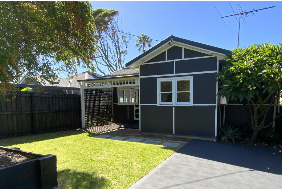
PHOTO SHOWING EXISTING COTTAGE TO BE DEMOLISHED
