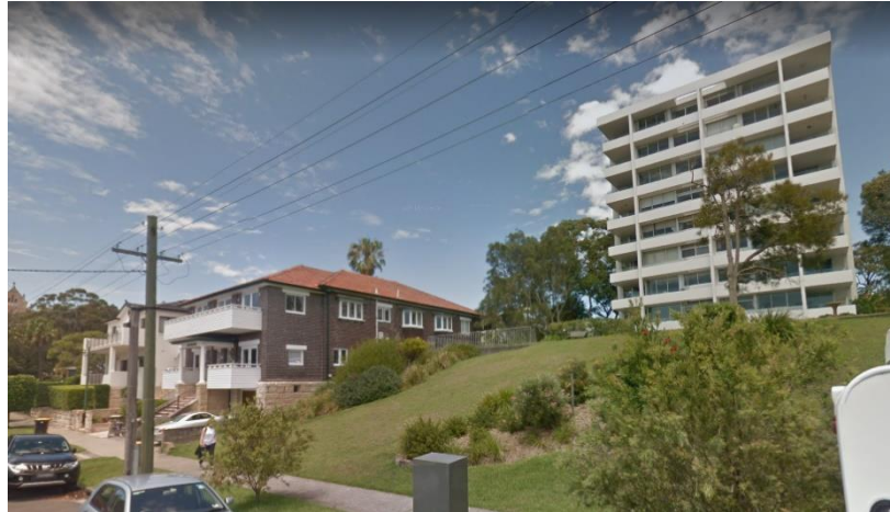
Figure 10: Mix of residential building typologies opposite the site fronting Reddall Street (Source: Google Maps)
