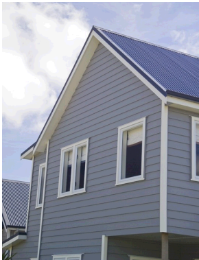
WINDOW TRIMS + ROOF FRAME: NON-COMBUSTIBLE TO COMPLY WITH BAL-40 Colour: White/Off Grey to match windows
