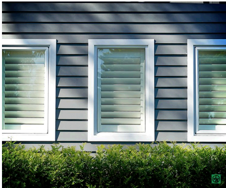
WINDOW TRIMS + ROOF FRAME: NON-COMBUSTIBLE TO COMPLY WITH BAL-40 Colour: White/Off Grey to match windows
