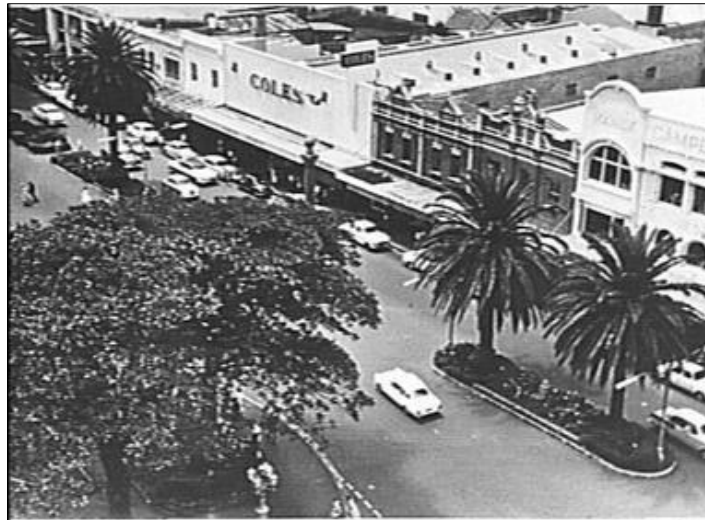
Figure 13: 1961 Image showing that the Emporium had been painted. The name “Campbells” remains visible on the centre panel of the parapet. Northern Beaches Council. Manly Local Studies Library.
