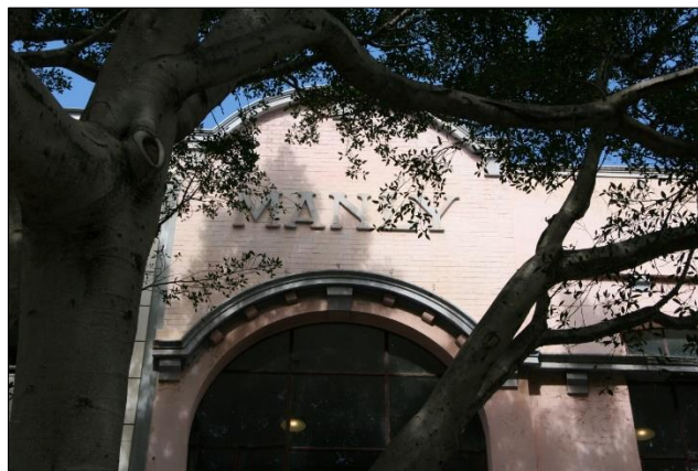
Figure 19: Detailing of the eastern parapet.
