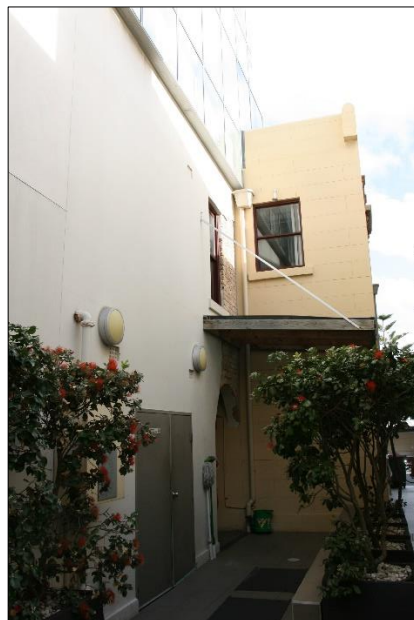
Figure 32: Image depicting the existing relationship between the rear wall of No.48 East Esplanade and the modern five storey mixed use commercial building.
