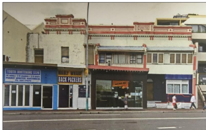
Figure 15: Appearance of No 46, 47 and 48 East Esplanade in 2008 prior to the restoration works. NBRS + Partners, Photographic Recording
