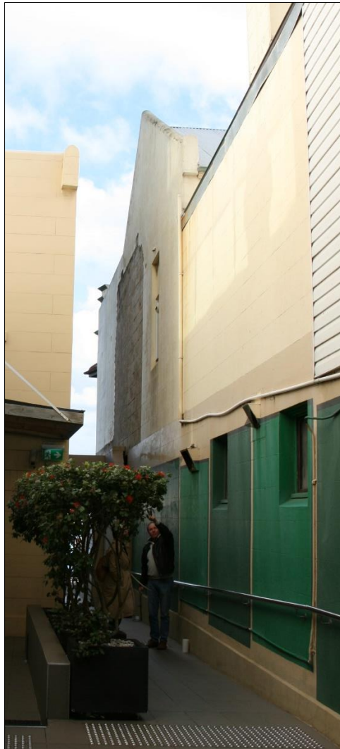
Figure 26: Details of the southern elevation of the laneway elevation.
