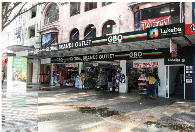
Figure 18: Detail of the ground floor of No. 6 The Corso.
