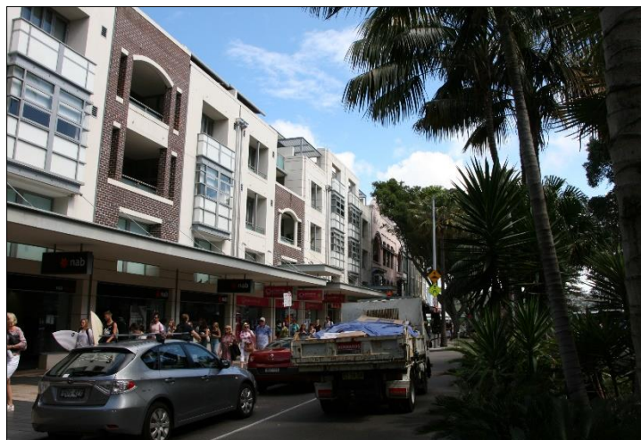
Figure 36: The modern adjoining development at Nos 8-28 The Corso.
