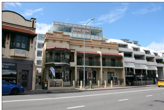
Figure 27: Nos 46-48 East Esplanade as viewed from the west.
