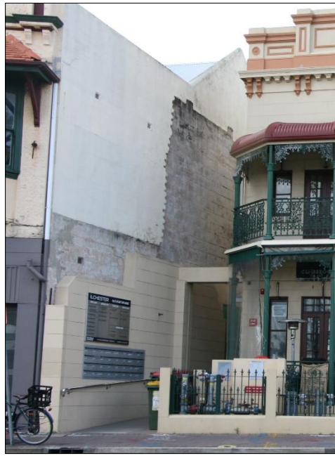
Figure 25: Detail of the laneway between No. 50 East Esplanade and No. 48 East Esplanade. The unpainted section of wall shows where the two buildings were previously attached.
