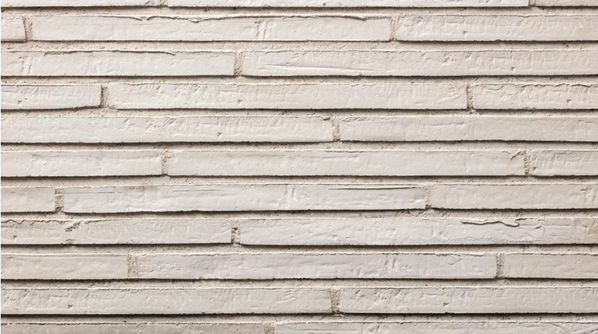
br brick walls
