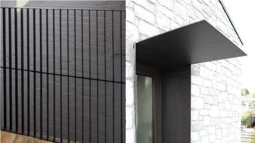
st steel balustrades, gates, fence + awning
