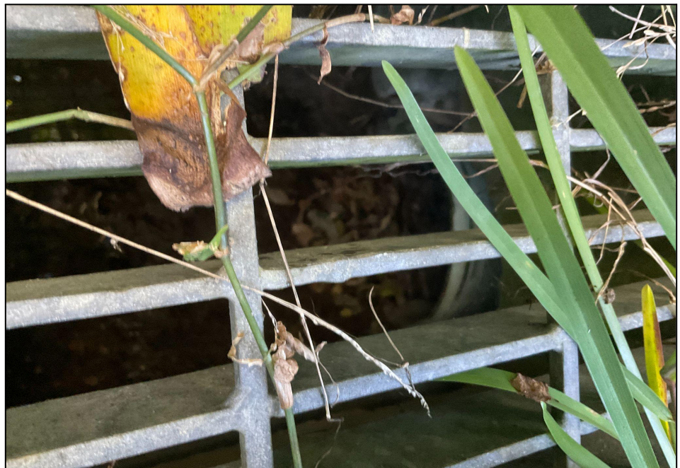
B4: Image of existing inter-allotment drainage pit within 16 Gertrude Avenue showing Ø300 P.V.C.
