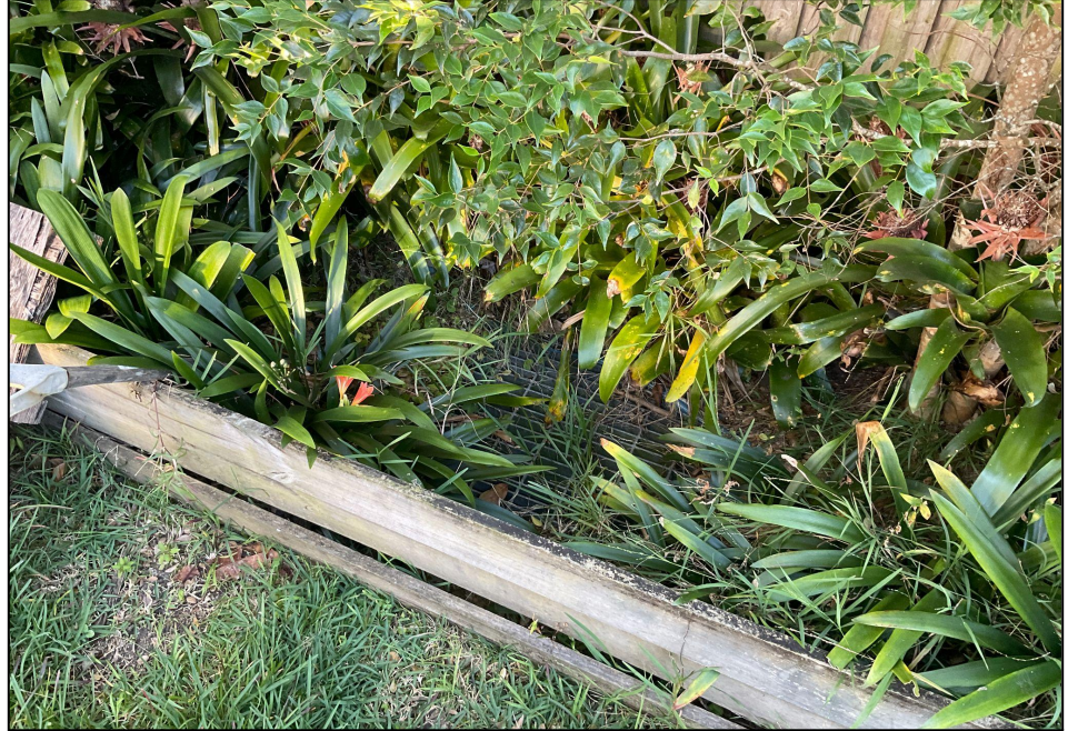
B3: Image of existing inter-allotment drainage pit within 16 Gertrude Avenue
