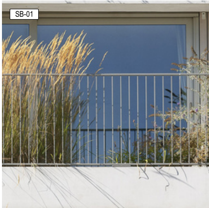
STEEL BALUSTRADE TO COMPLY WITH BCA
