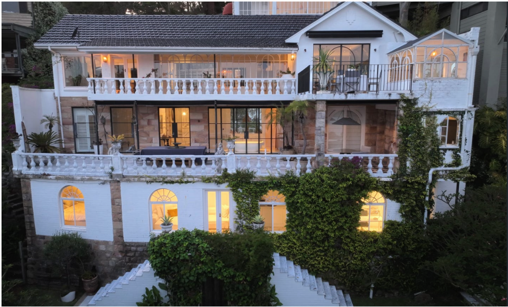
Rear View of Existing Dwelling
