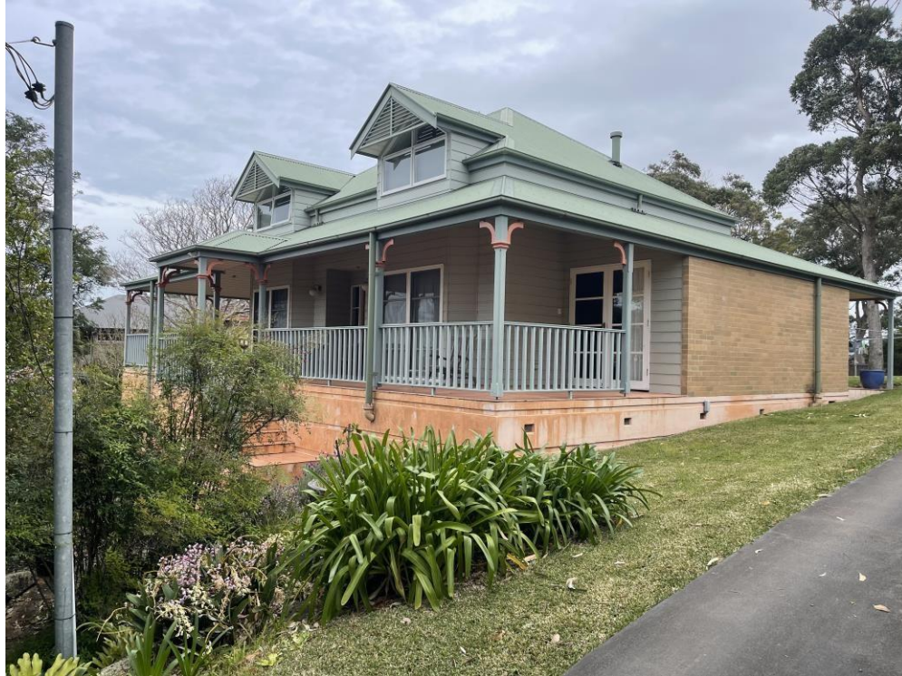
Fig 6: View of the subject dwelling, looking south-west from common access driveway towards location of proposed passing bay
