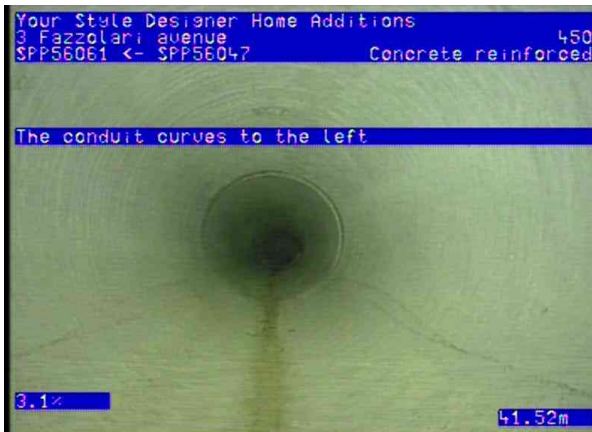
SPI50195_ee54ead3-a01f-40a8-bc6d-e162712ebe54_20250717_075503_204.jpg, 00:15:15, 41.52 The conduit curves to the left
