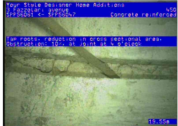
SPI50195_8f4c3fff-8801-47bd-8c30-f33521e3bfe9_20250717_074531_593.jpg, 00:06:56, 19.55 Tap roots, reduction in cross sectional area, Obstruction: 10%, at joint at 4 o'clock
