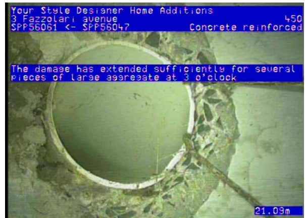
SPI50195_c70b843b-77fa-43cd-9401-9ed1842afa41_20250717_074627_748.jpg, 00:07:38, 21.09 The damage has extended sufficiently for several pieces of large aggregate at 3 o'clock
