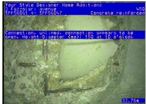
SPI50195_c57dc26f-6edf-4e3e-98ea-b8fa7592980f_20250717_075156_214.jpg, 00:12:24, 33.76 Connection, unlined, connection appears to be open, Height/Diameter (mm): 150 at 10 o'clock
