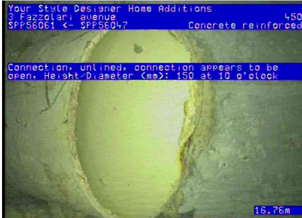
SPI50195_c4b506c8-7b9a-4194-82fb-1adf6b650383_20250717_074417_076.jpg, 00:05:48, 16.76 Connection, unlined, connection appears to be open, Height/Diameter (mm): 150 at 10 o'clock
