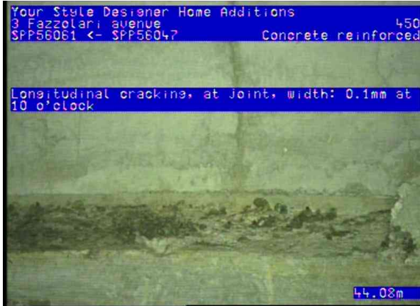
SPI50195_2649fa71-106a-47f7-971c-913f5edb0f2f_20250717_075637_532.jpg, 00:16:39, 44.08 Longitudinal cracking, at joint, width: 0.1mm at 10 o'clock
