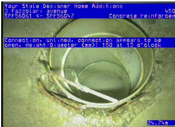
SPI50195_a12b57b7-9d0c-472e-825b-0966ac886c06_20250717_074858_918.jpg, 00:09:33, 24.74 Connection, unlined, connection appears to be open, Height/Diameter (mm): 150 at 12 o'clock
