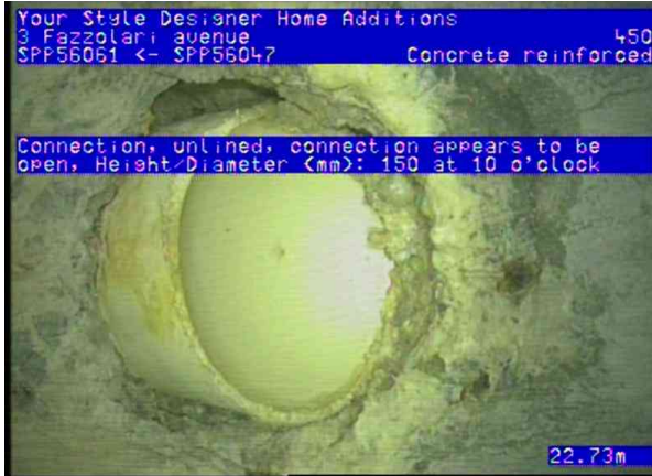
SPI50195_65d6a7c9-8581-4621-866b-a4aafc08ee69_20250717_074728_528.jpg, 00:08:33, 22.73 Connection, unlined, connection appears to be open, Height/Diameter (mm): 150 at 10 o'clock
