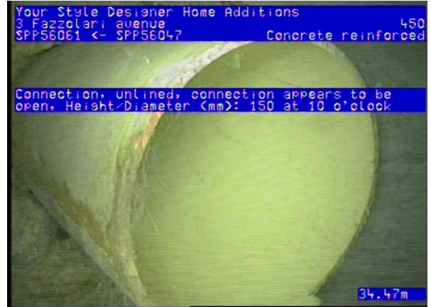
SPI50195_8ea5d1ed-199d-4735-98f3-bb28d7dcec5a_20250717_075256_013.jpg, 00:13:13, 34.47 Connection, unlined, connection appears to be open, Height/Diameter (mm): 150 at 10 o'clock
