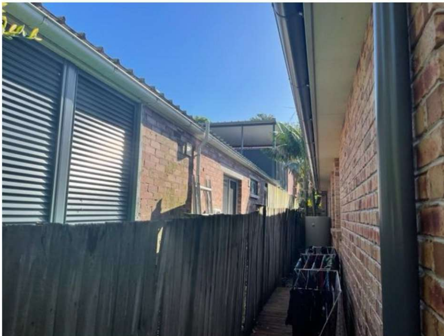
Photo 1-View facing east along the common side boundary
