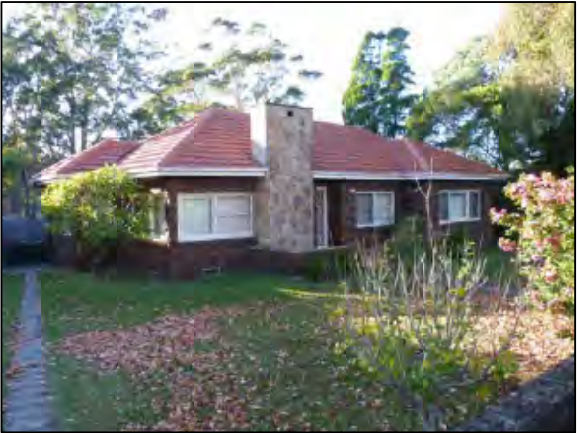
PHOTOGRAPH LOCATION 16 No.37 MELWOOD AVE
