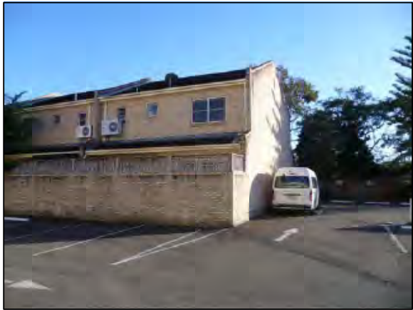
PHOTOGRAPH LOCATION 4 17-19 FORESTVILLE AVE
