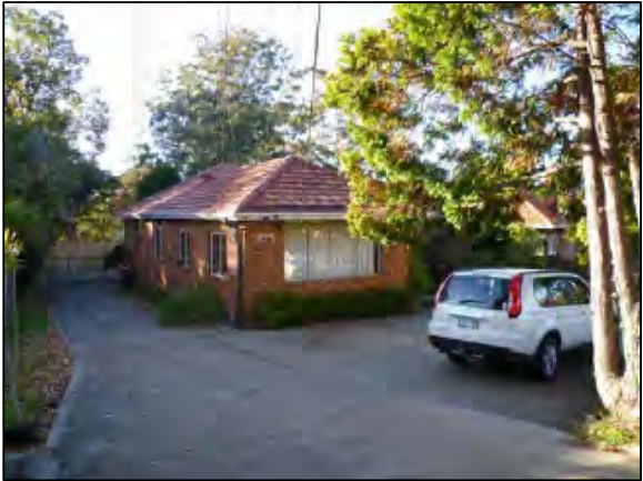
PHOTOGRAPH LOCATION 14 No.35 MELWOOD AVE
