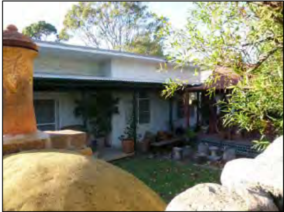
PHOTOGRAPH LOCATION 12 No.31 MELWOOD AVE
