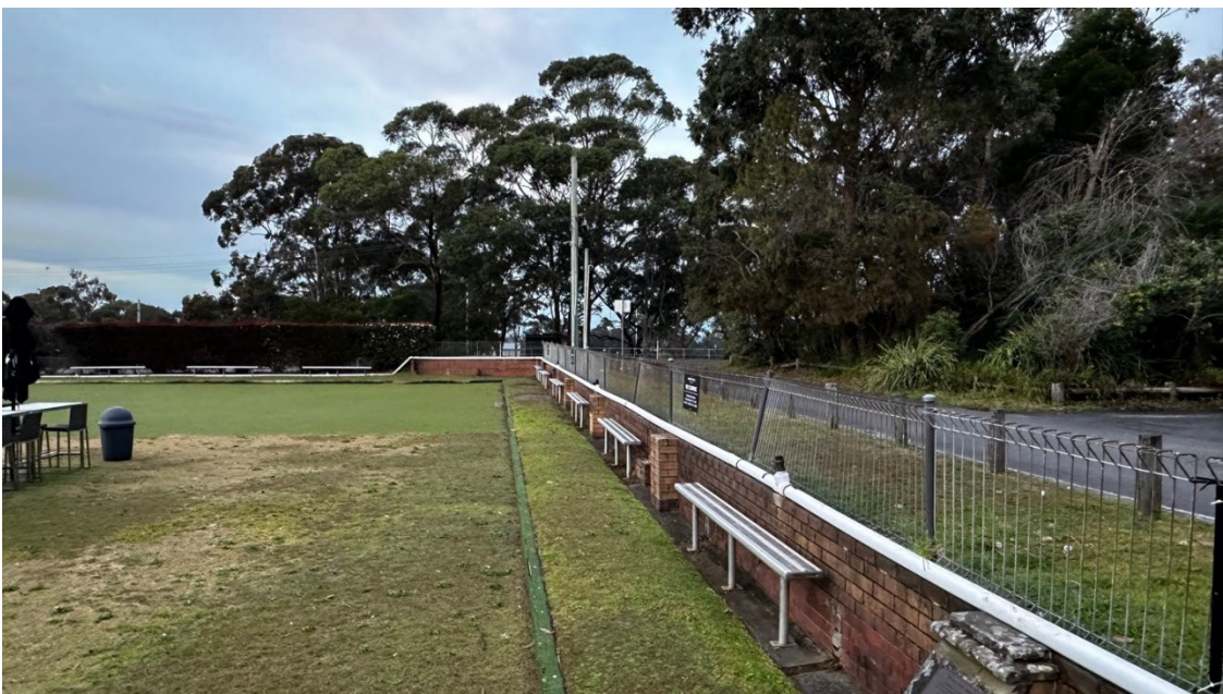
Plate 8 – View to the south, showing the low cut into the natural hillslope supported by a mortared brick retaining wall.
