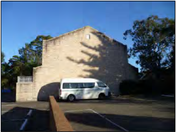
PHOTOGRAPH LOCATION 5 17-19 FORESTVILLE AVE
