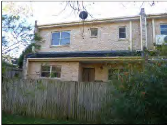
PHOTOGRAPH LOCATION 1 17-19 FORESTVILLE AVE
