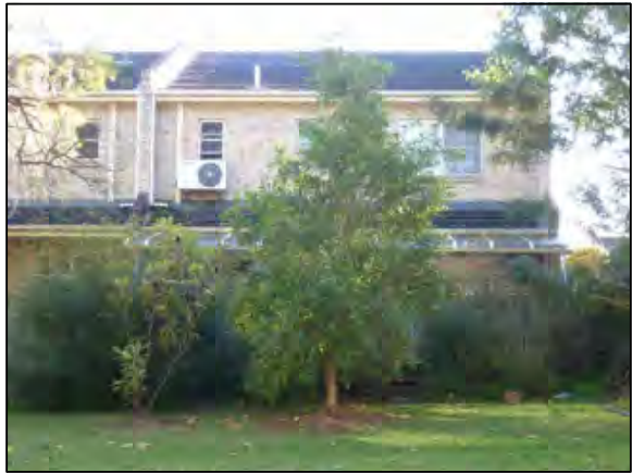
PHOTOGRAPH LOCATION 2 17-19 FORESTVILLE AVE
