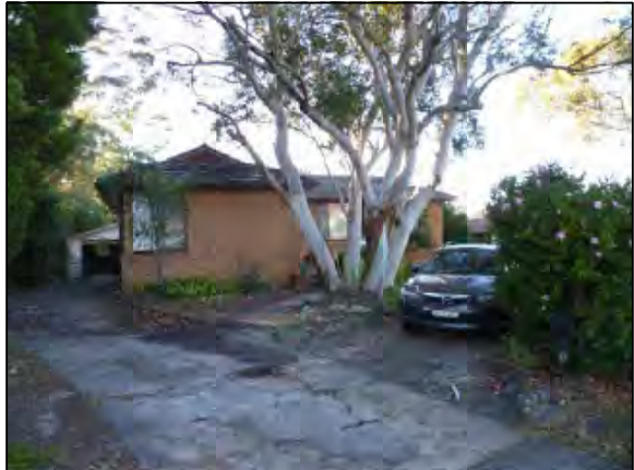
PHOTOGRAPH LOCATION 18 No.41 MELWOOD AVE
