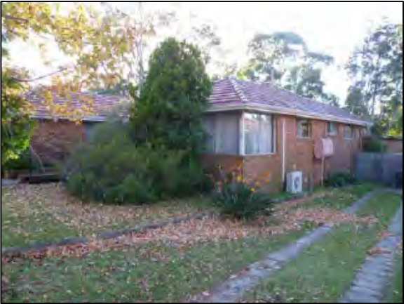
PHOTOGRAPH LOCATION 15 No.35 MELWOOD AVE
