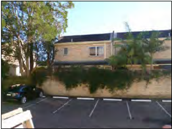
PHOTOGRAPH LOCATION 3 17-19 FORESTVILLE AVE
