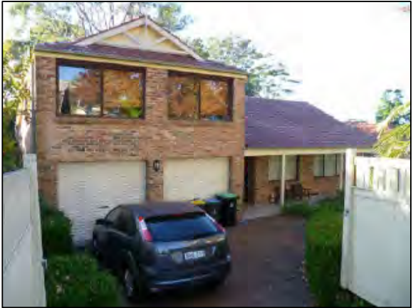
PHOTOGRAPH LOCATION 13 No.33 MELWOOD AVE
