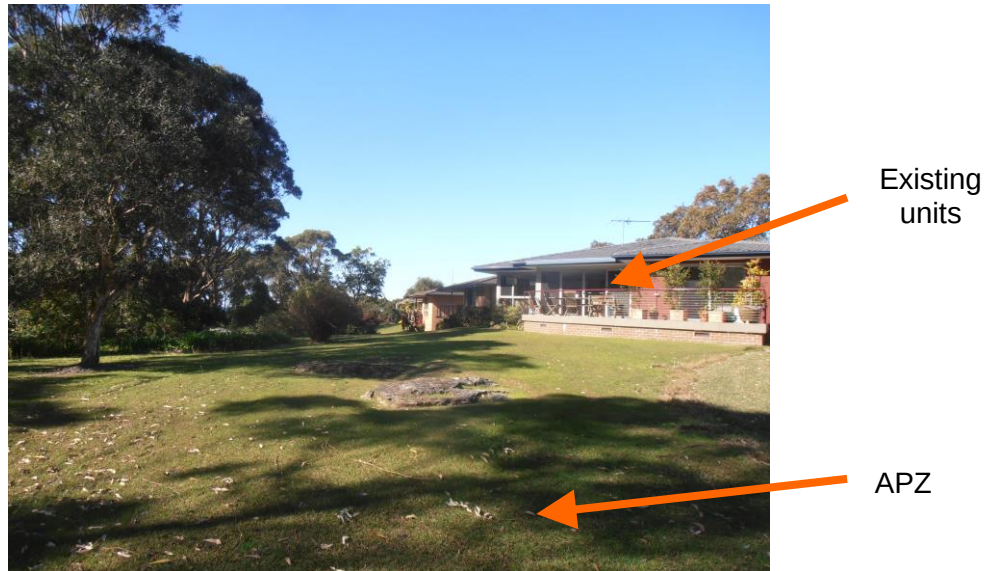
Photograph 04: View east along the existing APZ adjacent the subject units
