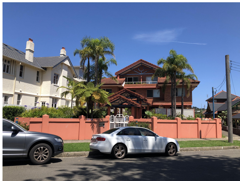
VIEW 1 - 22-26 ADDISON ROAD MANLY
