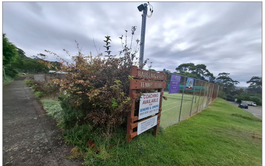
Subject site as viewed from Vista Avenue entry Source: GAT & Associates site inspection 26 th March 2025
