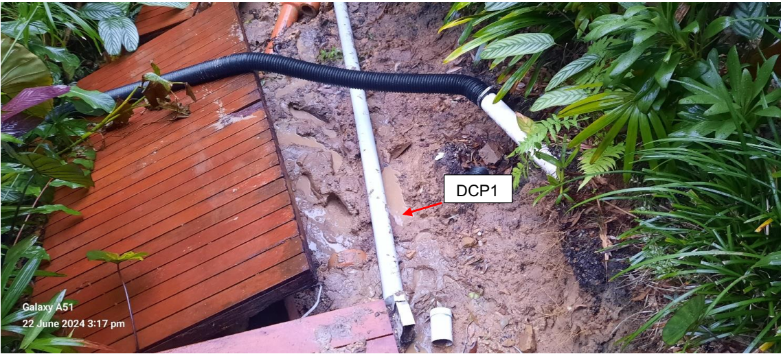
Plate 30: DCP1 test location, southern corner of concrete block, looking north-east.
