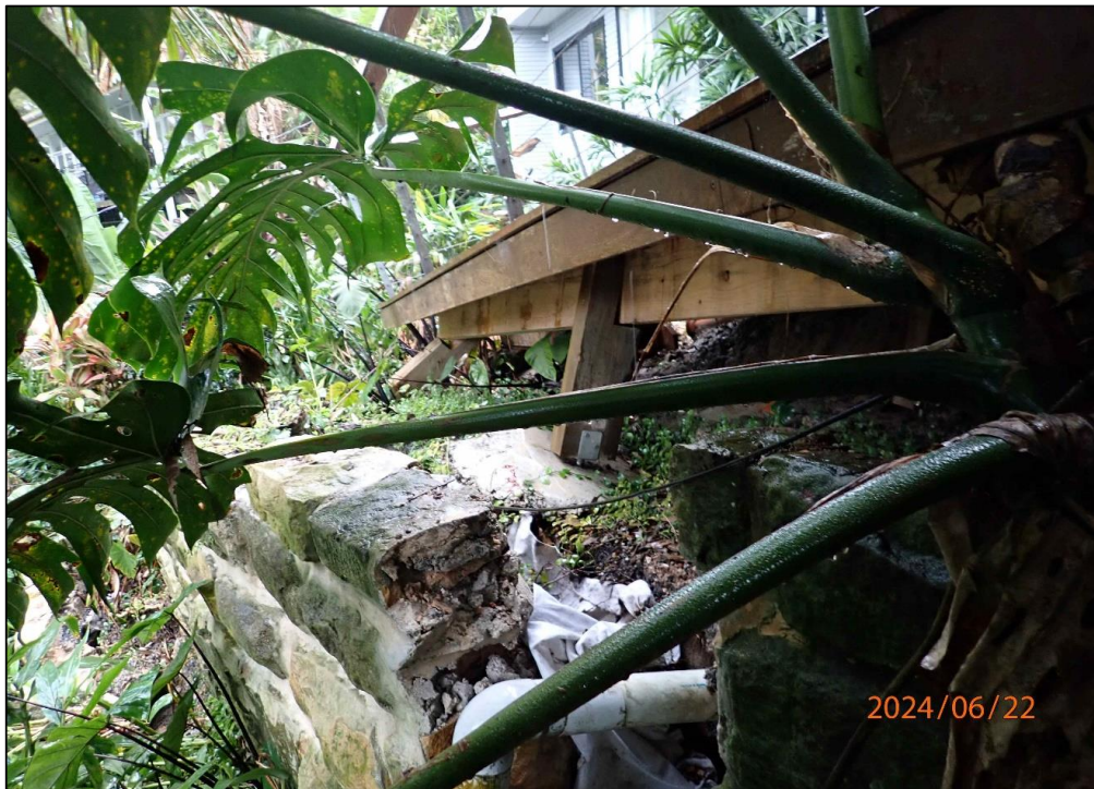
Plate 24: Timber post footings supported by concrete piles founded in colluvial soils, looking north.
