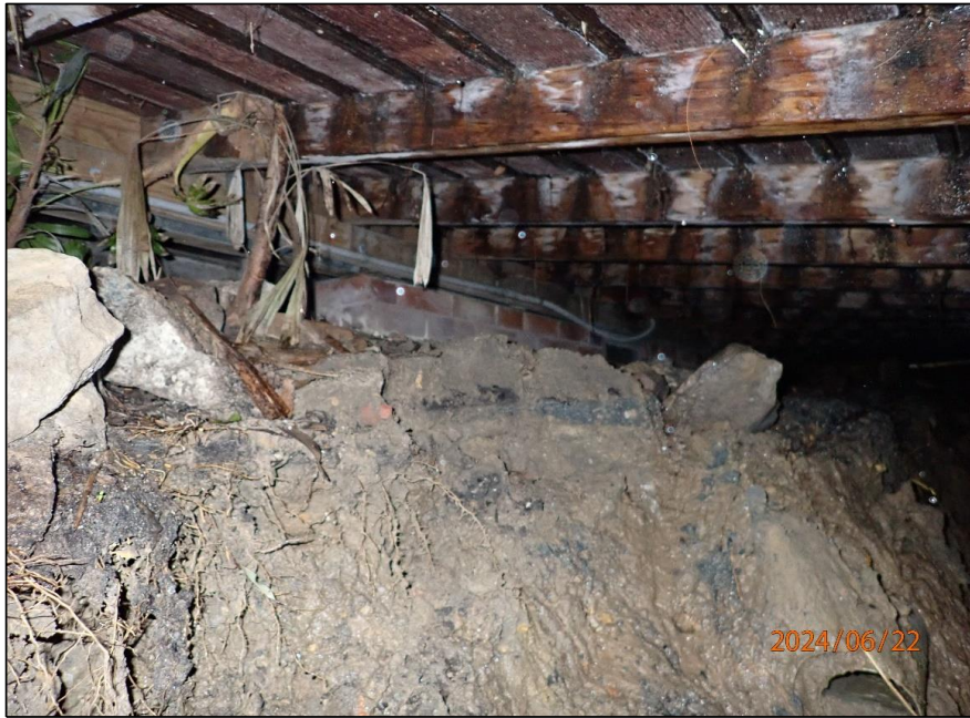
Plate 26: Saturated colluvium and boulders exposed underneath timber deck at LGF level, looking north-east.
