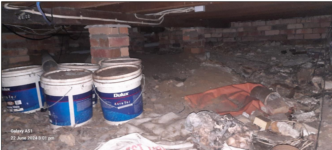
Plate 13: Strip and column footings supporting the upper floor level, looking south.
