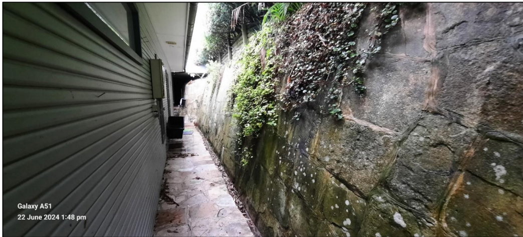
Plate 11: Stone paved pathway and stone wall along western side of upper floor level, looking south.
