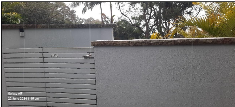
Plate 6: Access door through rear eastern boundary of No. 46, leading to No. 46A, looking east.
