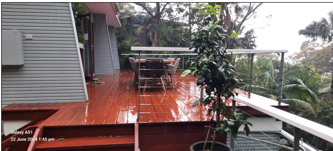
Plate 9: Raised timber deck located to east of upper floor level, looking north.
