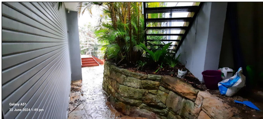
Plate 12: Stone paved pathway and stairway/stone wall along southern side of upper floor level, looking east.
