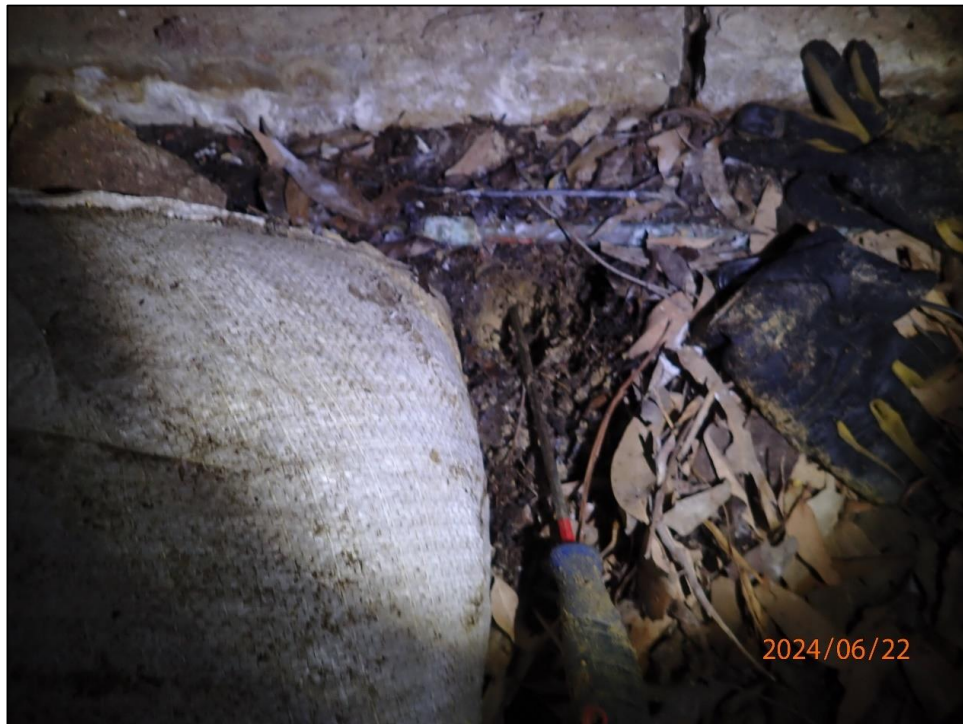
Plate 28: Concrete pad of brick strip footing founded on colluvium, looking west.
