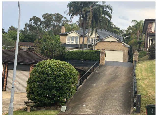
Street View of 105 John Oxley Drive
