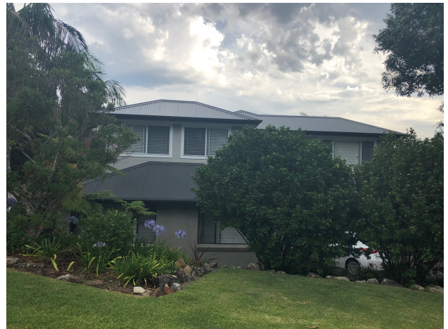
Street View of 104 John Oxley Drive
