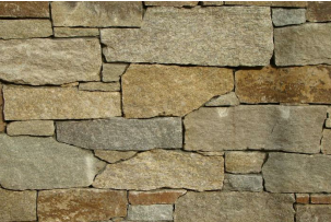
SANDSTONE FINISH TO RET. WALLS
