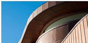
G - COPPER STYLE ROOFING
