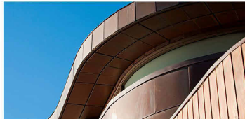
G - COPPER STYLE ROOFING
