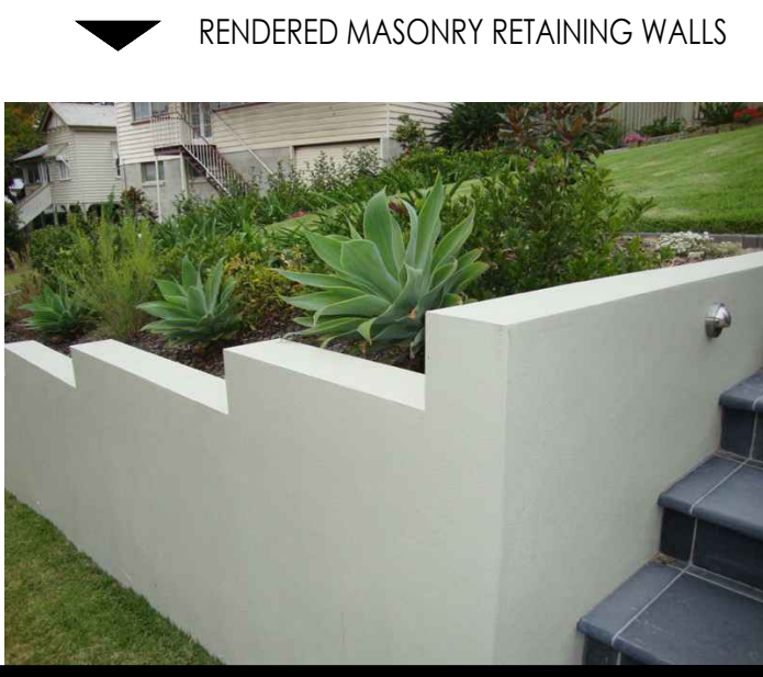
RENDERED MASONRY RETAINING WALLS
