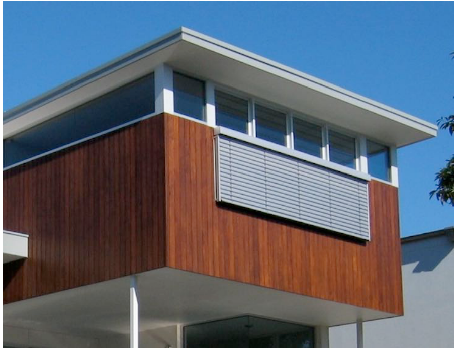
TC Timber cladding wall, colour: natural, with external blind to window
