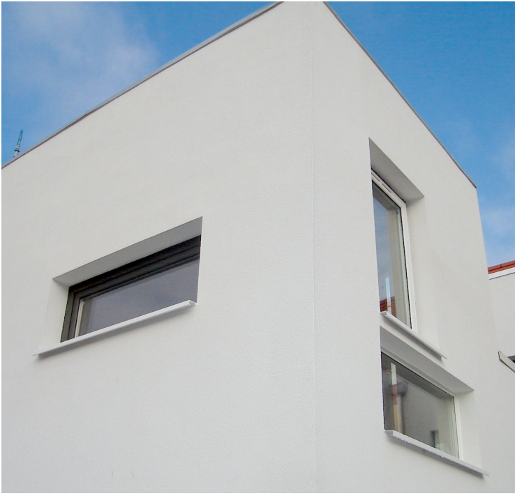
RW Rendered masonry wall painted finish colour : Light
