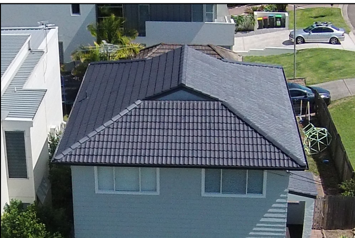
TILED ROOF & DUTCH GABLE TO MATCH EXISTING
