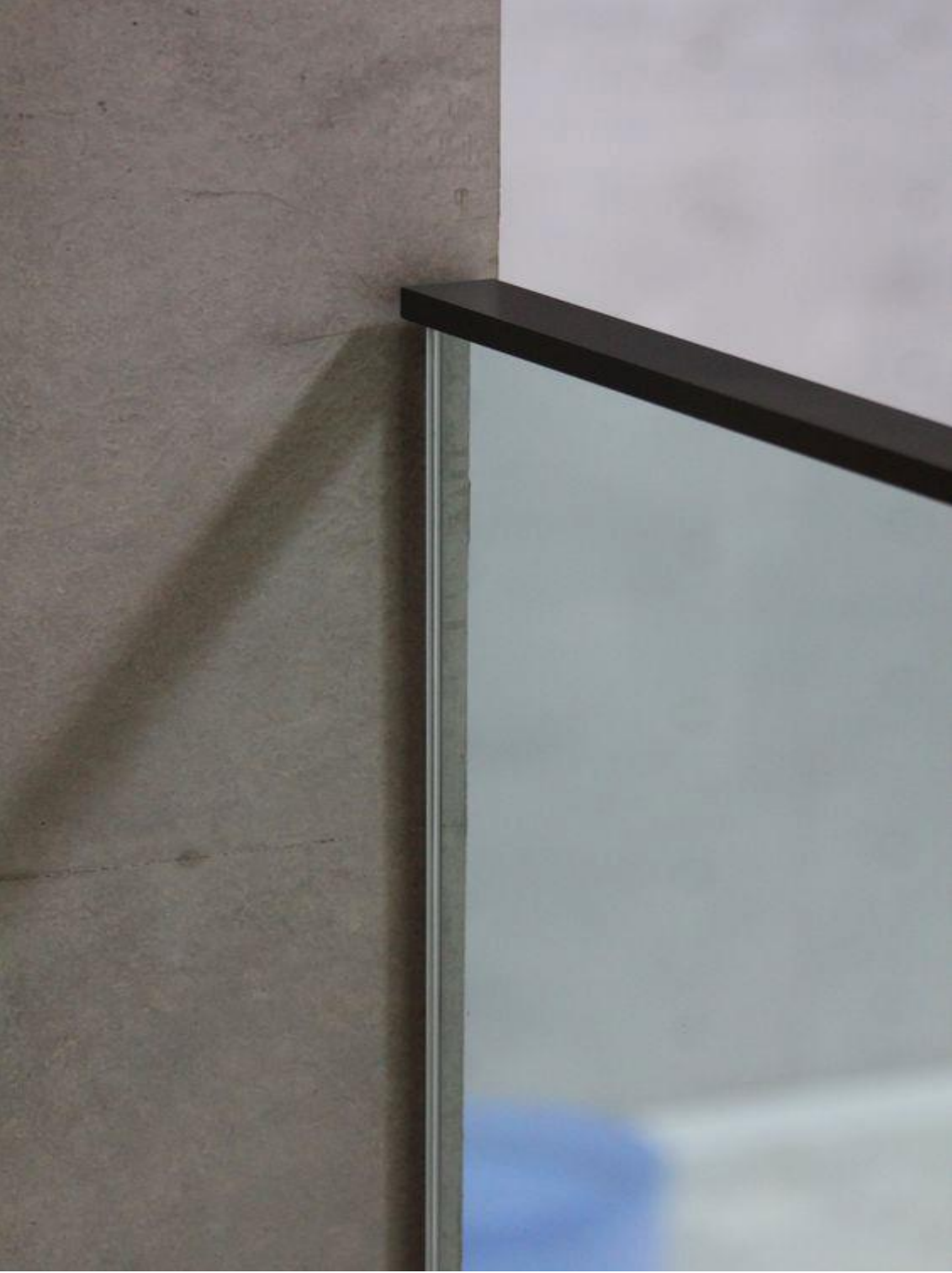
4 FRAMELESS GLASS BALUSTRADE WITH BRONZE CAPPING
