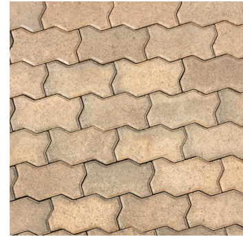
EXISTING STREET PAVING INTERLOCKING BRICK PAVERS
