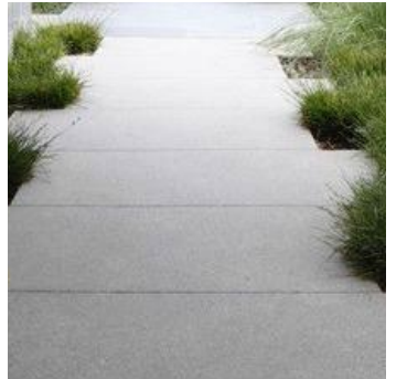
PROPOSED COURTYARD PAVING CONCRETE PAVERS, LARGE FORMAT
