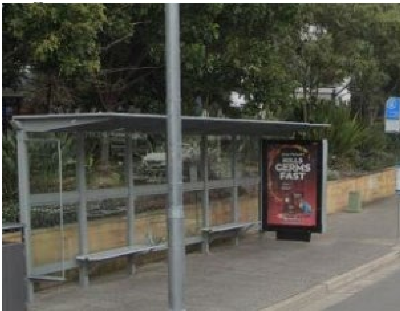
Figure 9: View of Shelter J7 and Advertising Signage Panel
