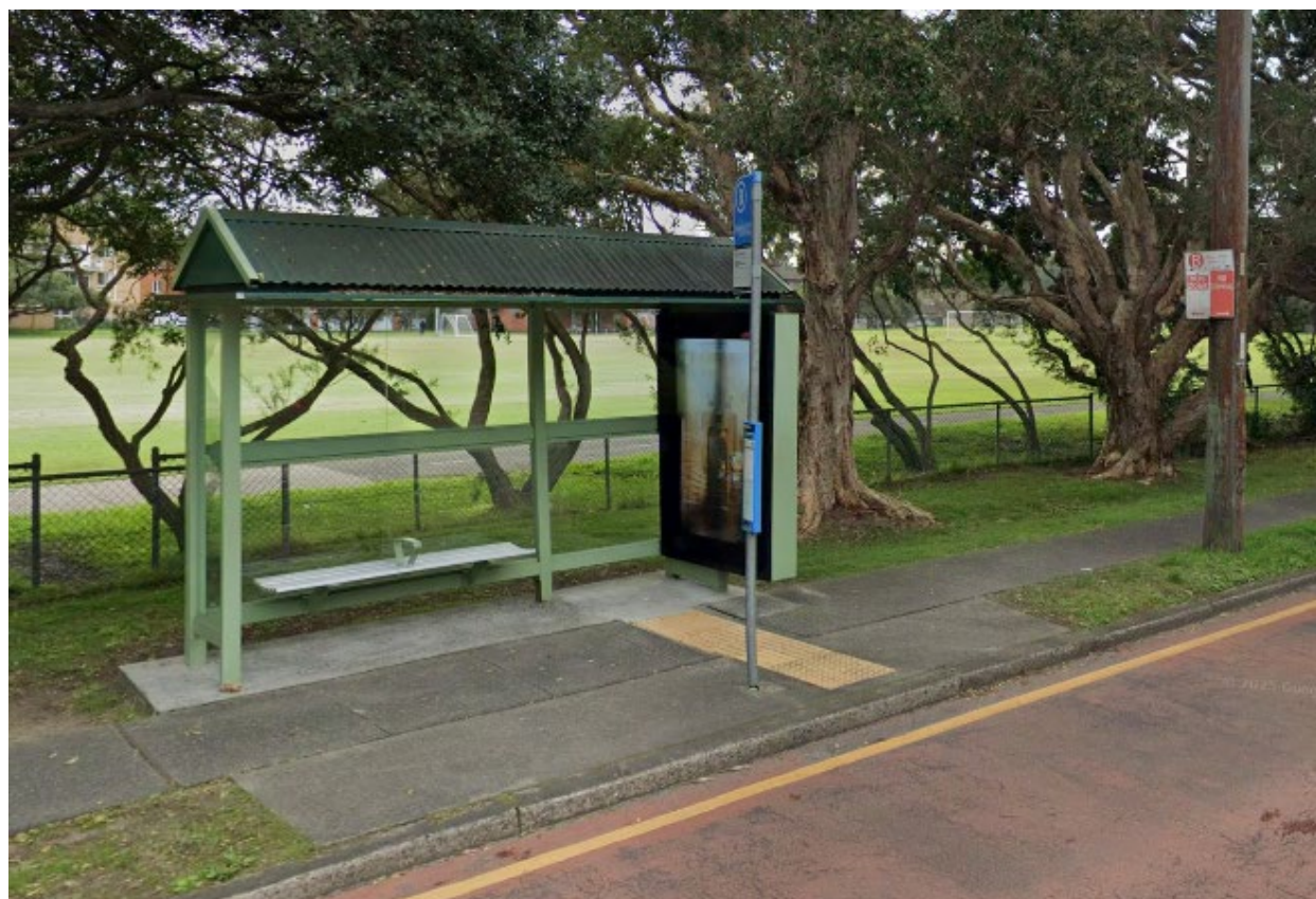
Figure 5: View of Shelter J2 and Advertising Signage Panel
