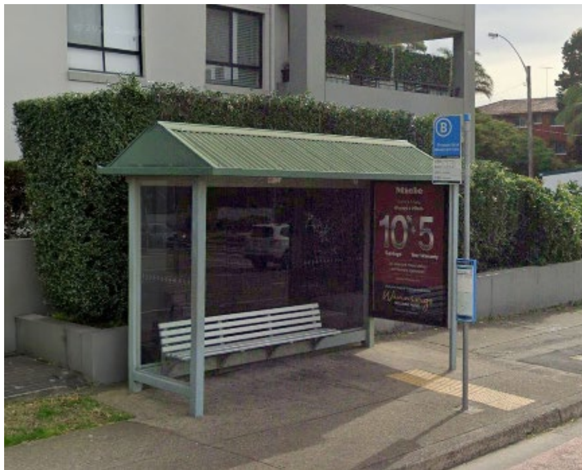
Figure 3: View of Shelter J1 and Advertising Signage Panel from Pittwater Road
