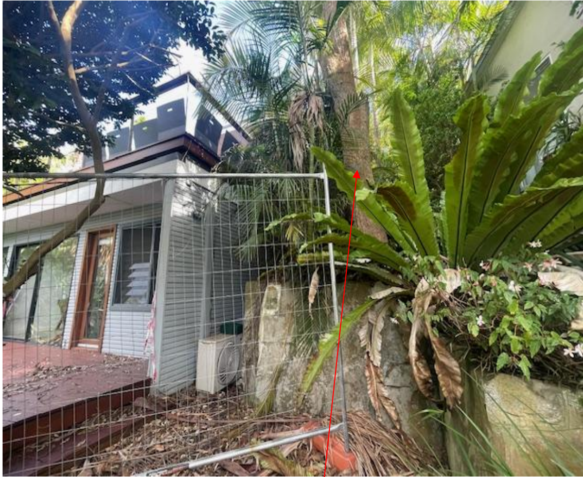
Photo A: The Looking from the lower ground floor at Tree 3 which is contained within a stone planter and will not be impacted by the associated encroachment of the deck.
