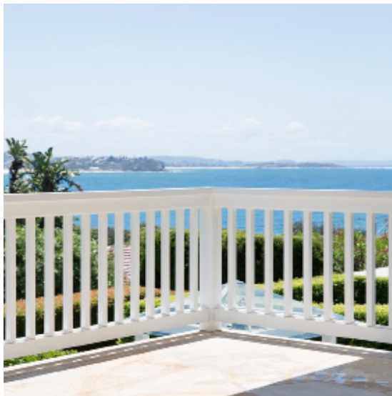
5. White Painted Timber Balustrading
