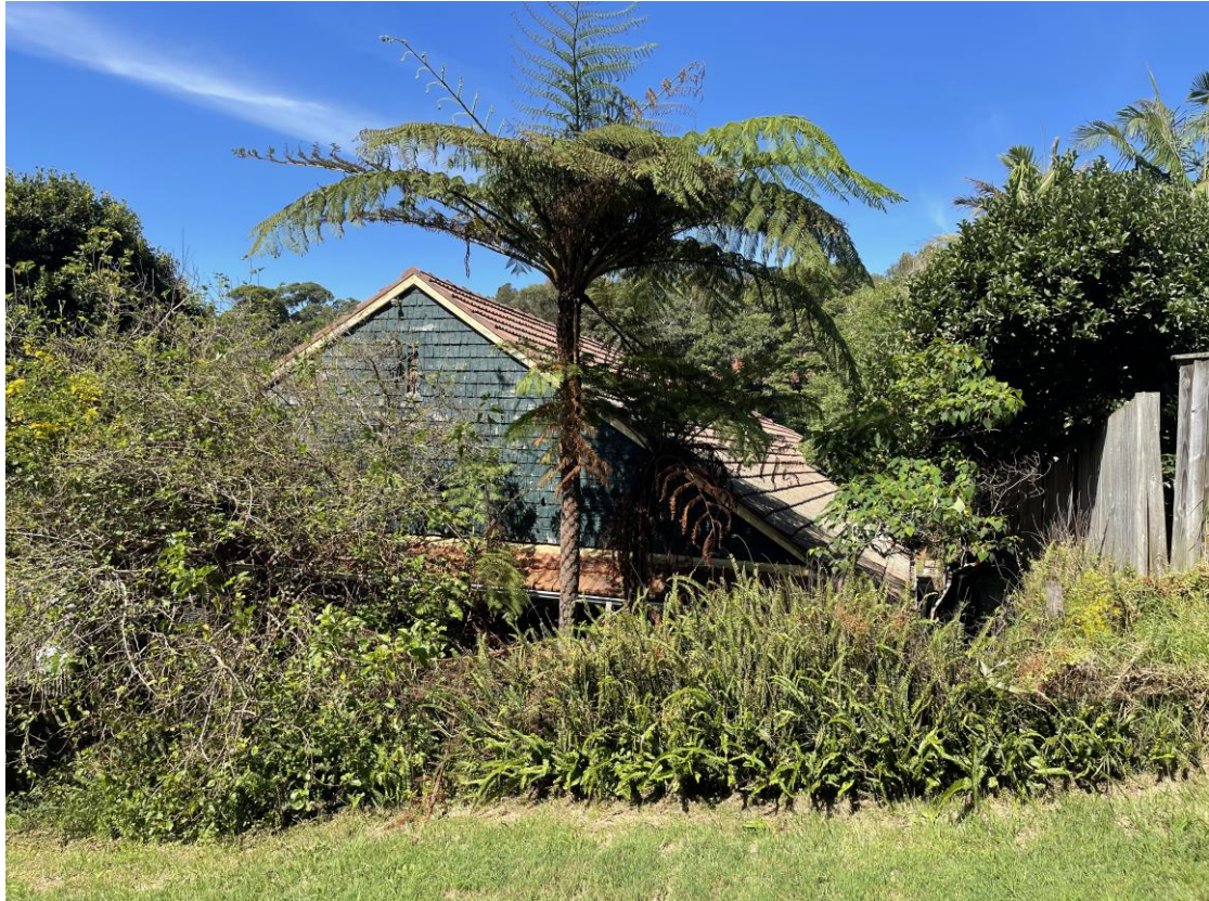
Fig 6: View of the subject dwelling, looking east from the adjacent public walkway
