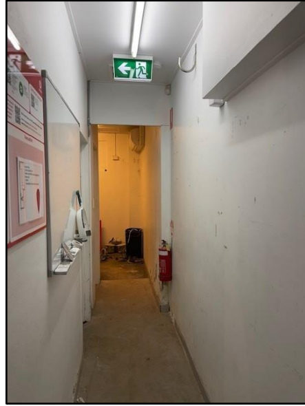
Figure 35. Interior view of rear hallway, facing south. (Source: Heritage 21)
