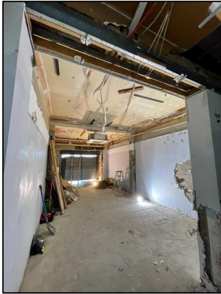
Figure 30. Interior view of the ground floor commercial space, facing north towards the Corso. (Source: Heritage 21)
