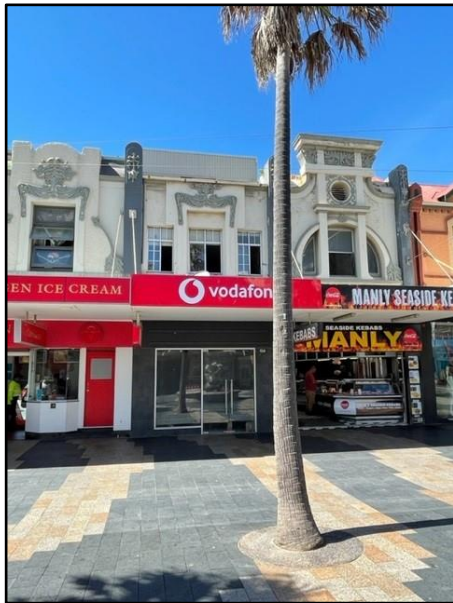
Figure 26. Exterior façade of commercial shop front facing south from the Corso highlighting Federation and Art Nouveau architectural detail amongst cluster. (Source: Heritage 21)
