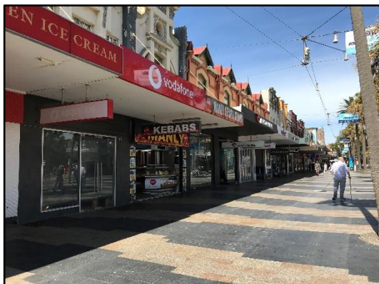
Figure 28. External view of the cantilevered awning along the Corso facing southwest. (Source: Heritage 21)
